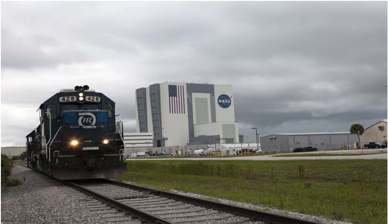
A Florida East Coast Railway locomotive rolling past the Vehicle Assembly Building at KSC
