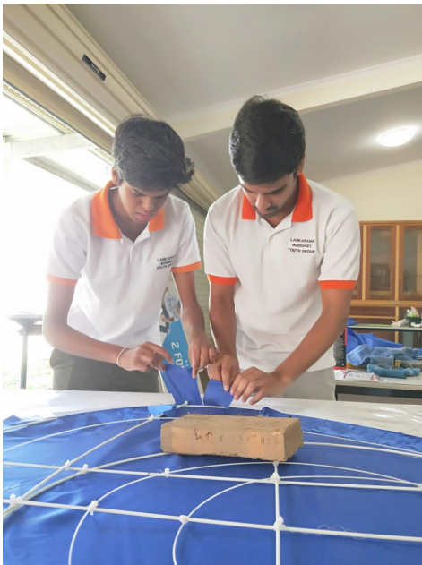
Gluing the blue silk satin fabric over the tail's fibreglass frame.
