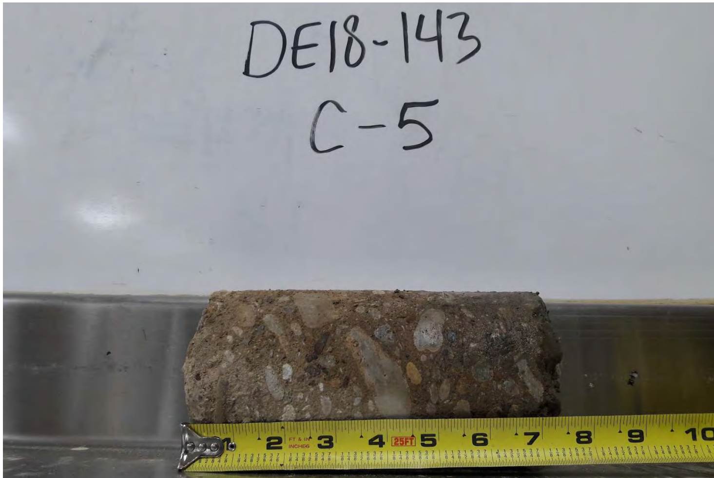
Photo 10: Photo of Pavement Core at Boring C-5.
