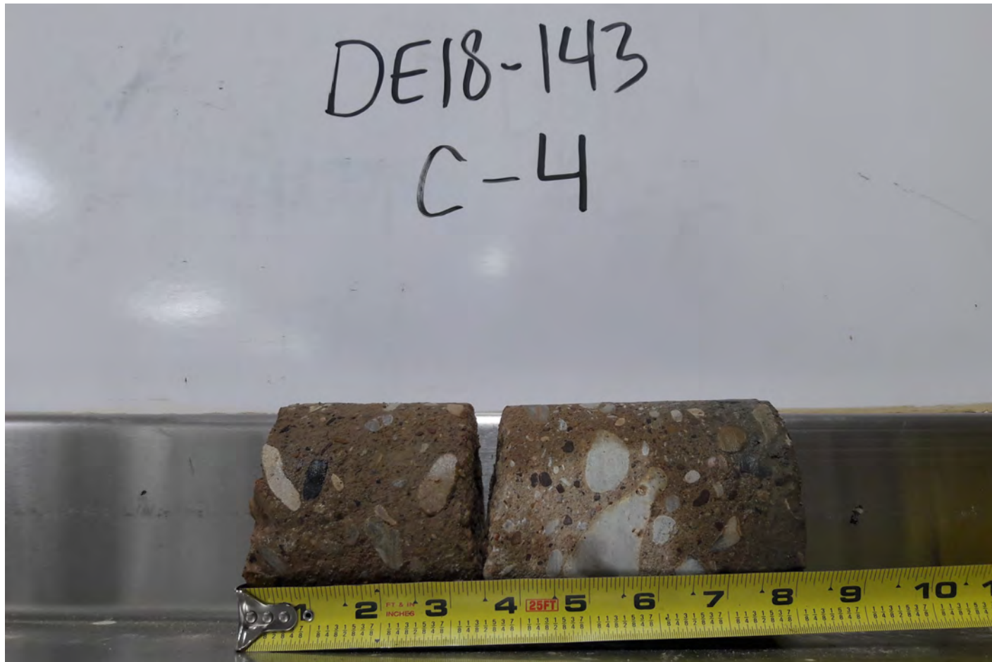
Photo 8: Photo of Pavement Core at Boring C-4.
