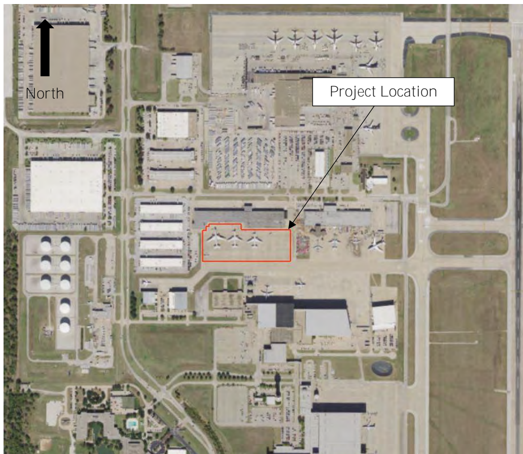
Figure 1 Overview of Evergreen Cargo Ramp
