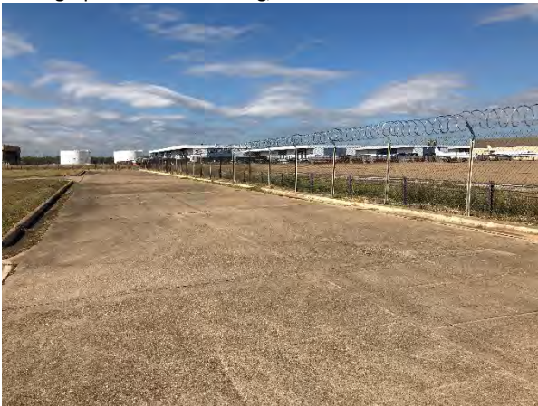
Photograph 13 – KHA Building, View to the West
