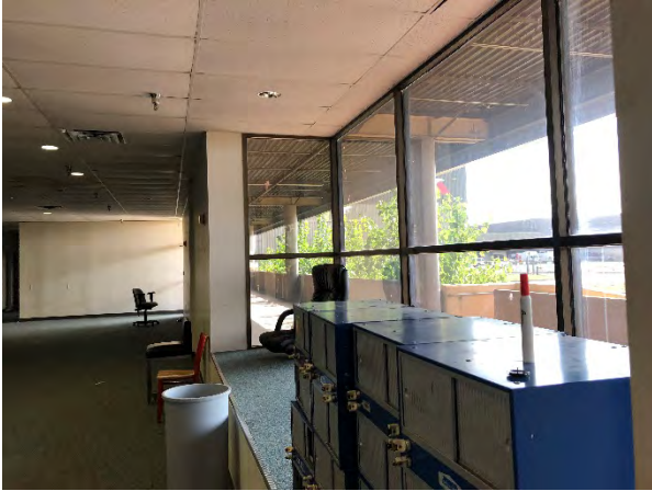
Photograph 19 – KHA Building, Interior
