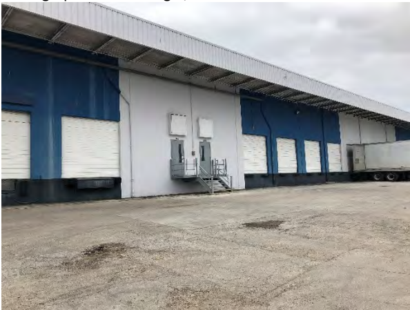
Photograph 37 – Building B, View to the South
