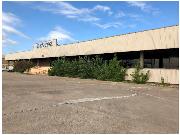
Photograph 2 – KHA Building, View to the Northwest
