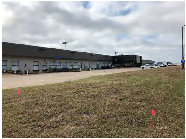
Photograph 2 - Evergreen Facility, View to the Southwest
