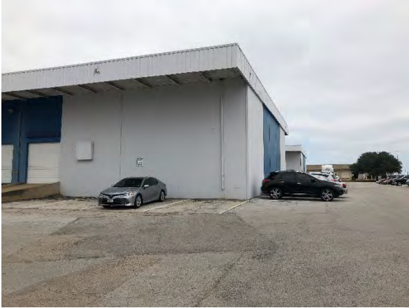
Photograph 35 – Building B, View to the North
