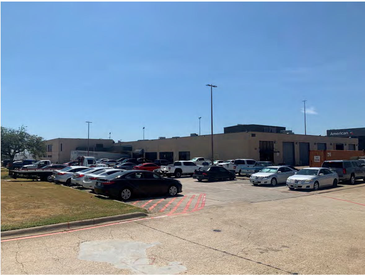
Photograph 1: American Airlines West Warehouse, north and west elevations, facing southeast.
