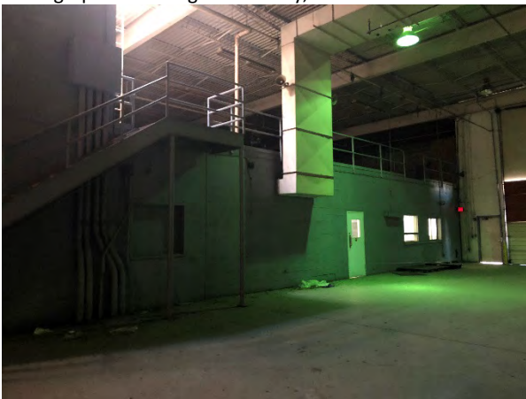
Photograph 21 – Evergreen Facility, Interior
