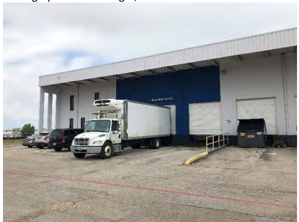
Photograph 64 – Building D, View to the North
