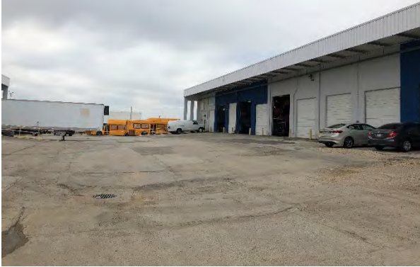
Photograph 51 – Building C, View to the Northwest
