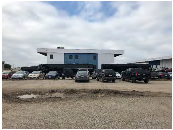
Photograph 66 – Building D, View to the West
