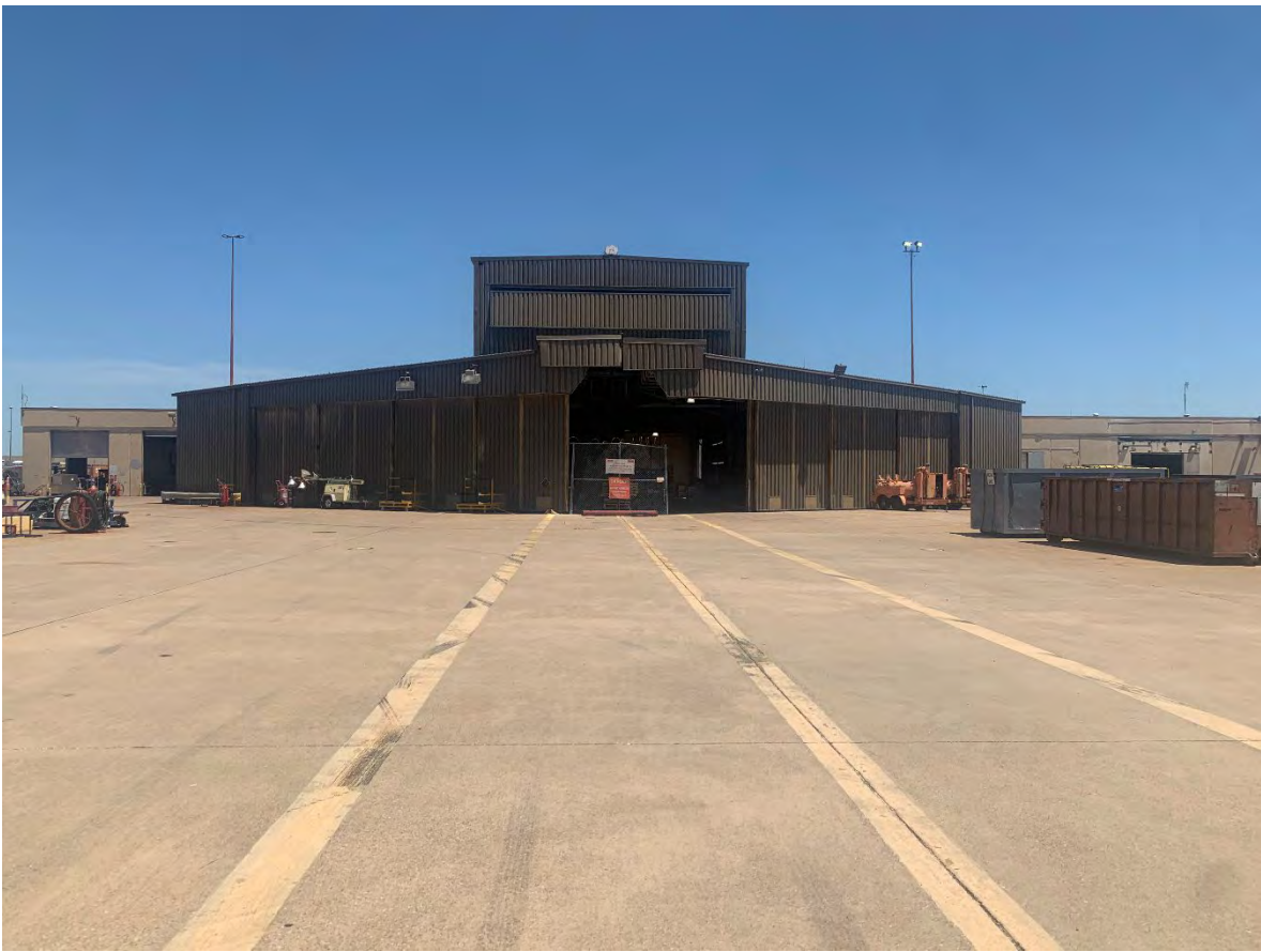
Photograph 15: American Airlines West Warehouse, south (western section) elevation, facing north.
