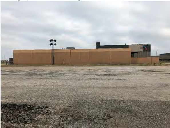
Photograph 7 – KHA Building, View to the East
