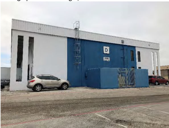
Photograph 23 – Building D, View to the East
