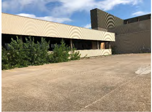
Photograph 4 – KHA Building, View to the Northeast
