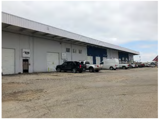
Photograph 50 – Building C, View to the Southeast
