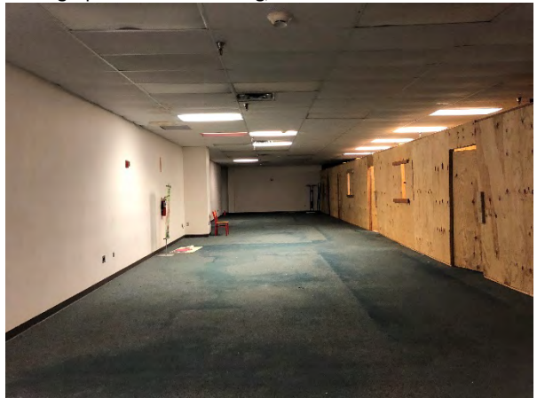
Photograph 16 – KHA Building, Interior
