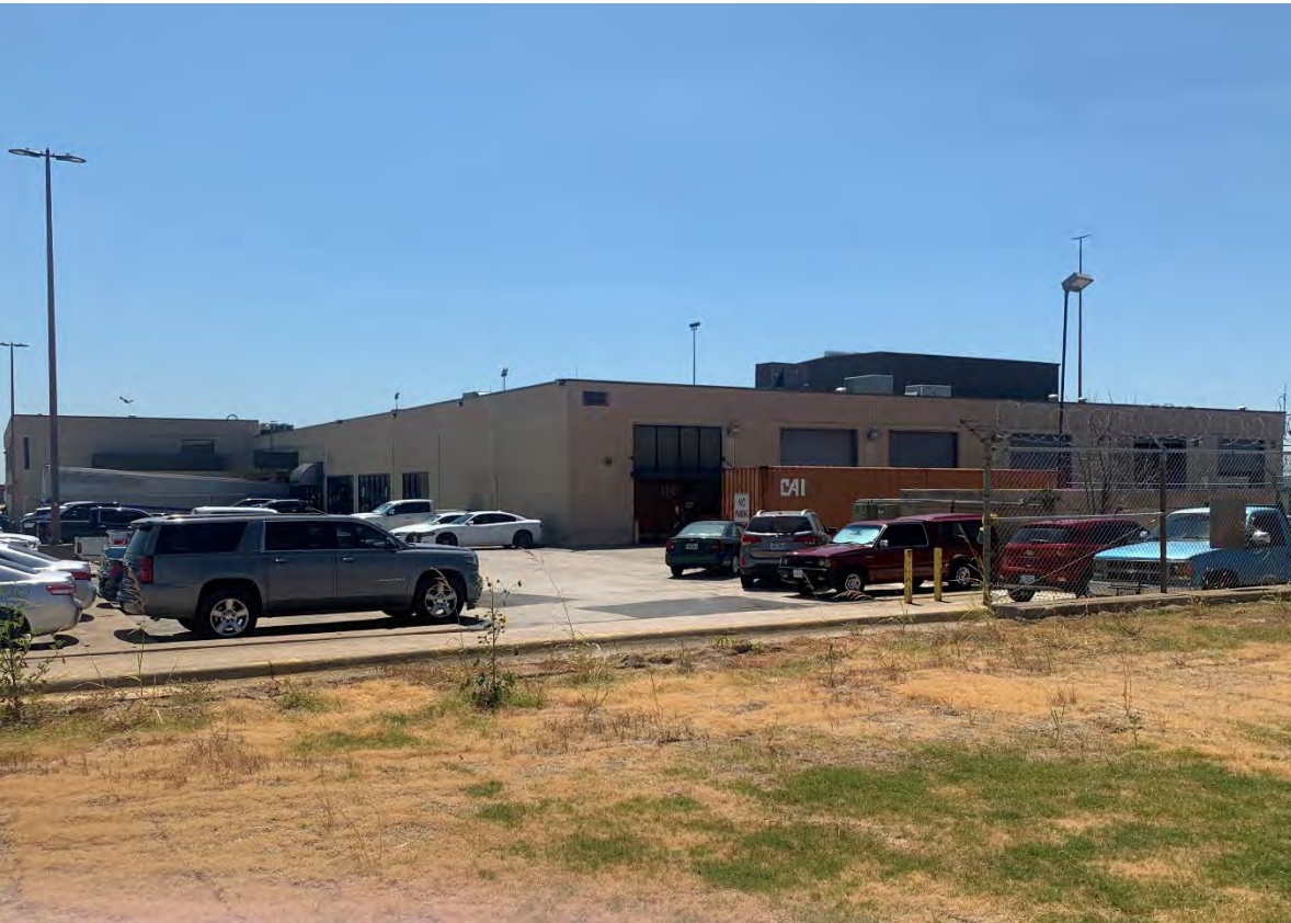
Photograph 2: American Airlines West Warehouse, north and west elevations, facing east.
