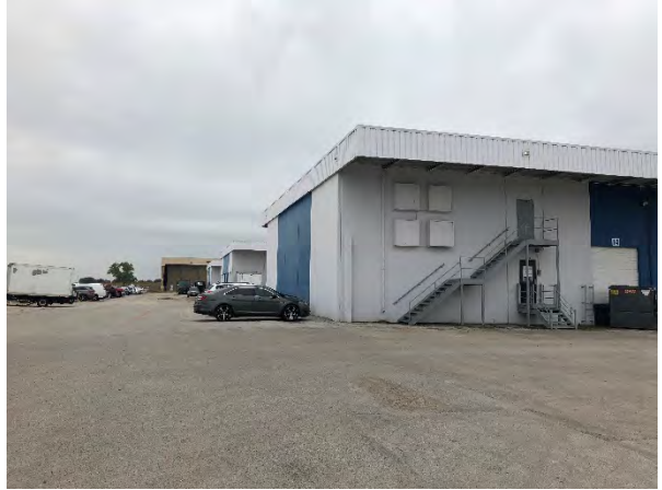
Photograph 36 – Building B, View to the South
