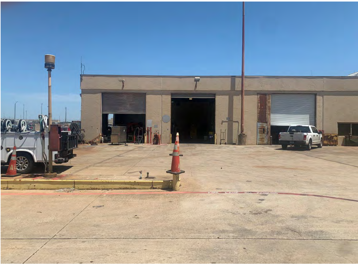
Photograph 19: American Airlines West Warehouse, south (western section) elevation, facing north.
