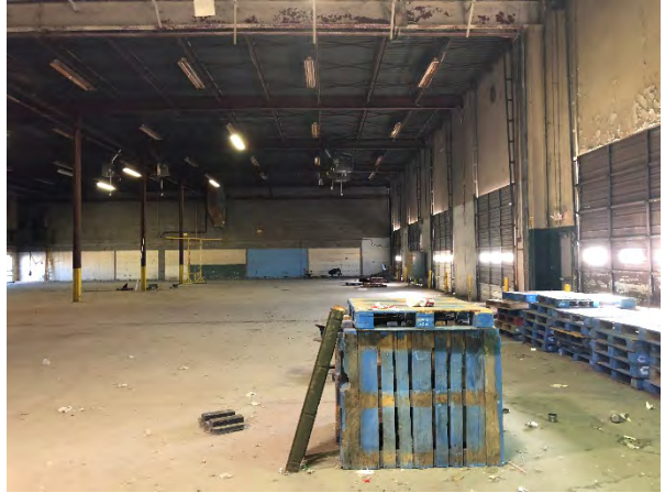
Photograph 20 – Evergreen Facility, Interior
