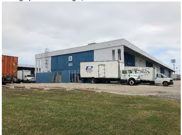
Photograph 32 – Building B, View to the Northeast
