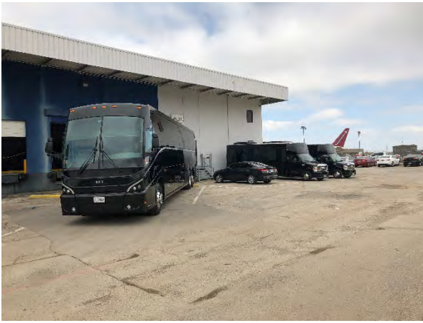
Photograph 65 – Building D, View to the Northeast
