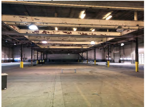
Photograph 14 - Evergreen Facility, Interior
