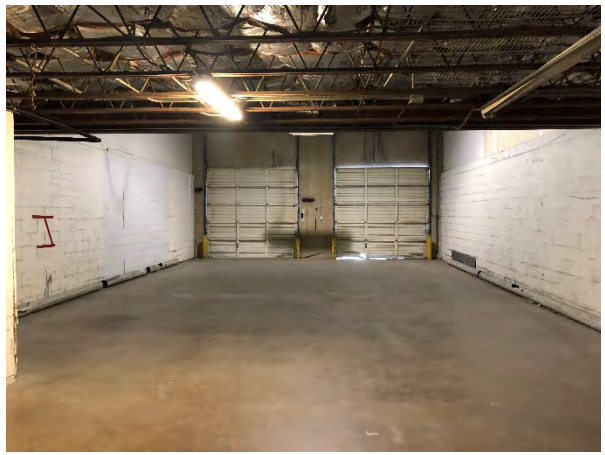
Photograph 58 – Building C, Interior
