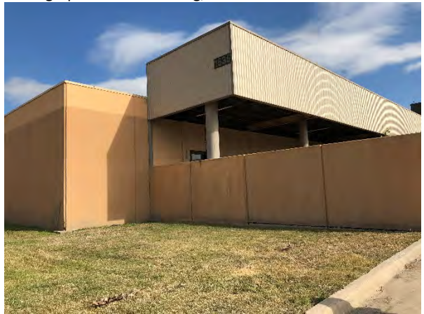
Photograph 6 – KHA Building, View to the Northeast
