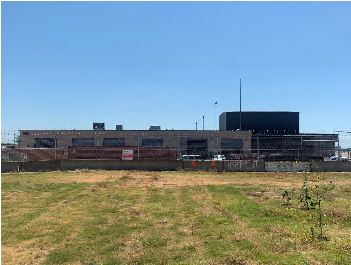
Photograph 3: American Airlines West Warehouse, west elevation, facing east.
