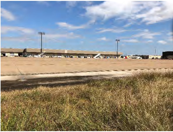
Photograph 9 - Evergreen Facility, View to the Northeast
