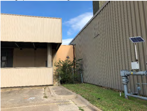
Photograph 5 – KHA Building, View to the North
