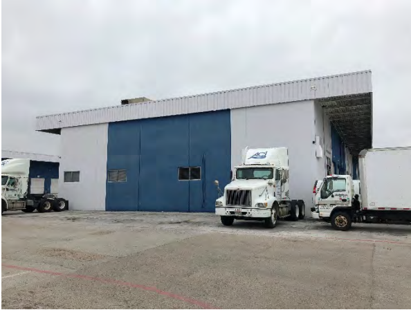
Photograph 27 – Building A, View to the West
