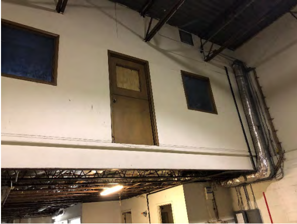
Photograph 59 – Building C, Interior
