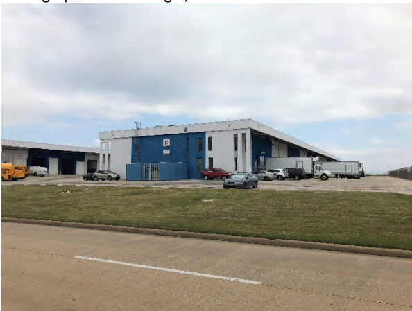
Photograph 63 – Building D, View to the Northeast
