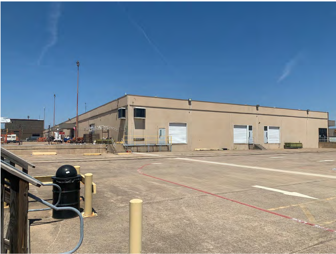
Photograph 11: American Airlines West Warehouse, south and east elevations, facing northwest.
