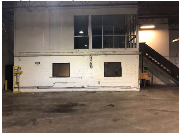
Photograph 56 – Building C, Interior
