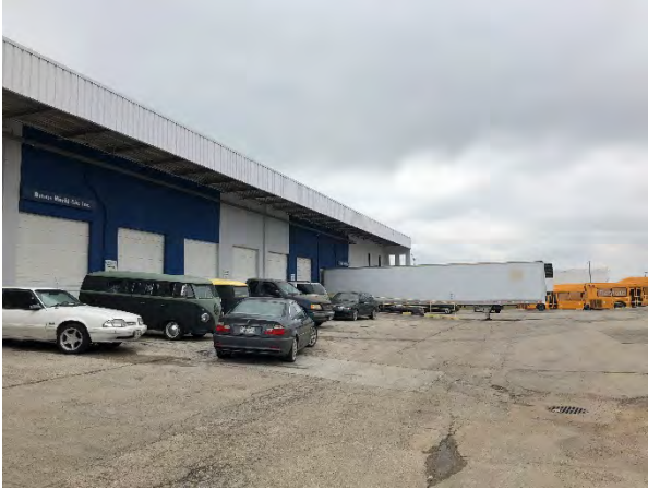
Photograph 67 – Building D, View to the Southeast
