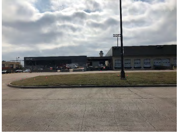
Photograph 12 - Evergreen Facility, View to the South
