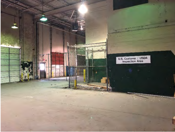
Photograph 19 – Evergreen Facility, Interior
