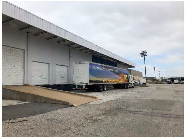
Photograph 34 – Building B, View to the Northeast
