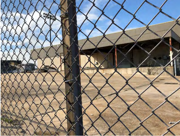
Photograph 11 - Evergreen Facility, View to the West
