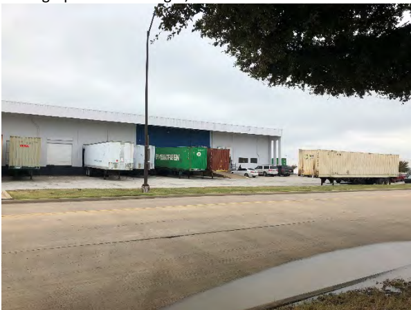
Photograph 29 – Building A, View to the South
