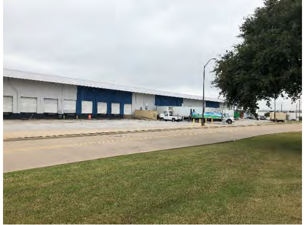
Photograph 28 – Building A, View to the South
