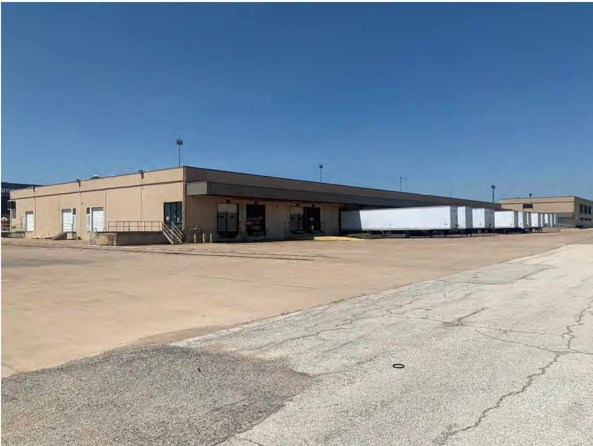
Photograph 8: American Airlines West Warehouse, north and east elevations, facing southwest.
