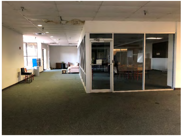
Photograph 18 – KHA Building, Interior
