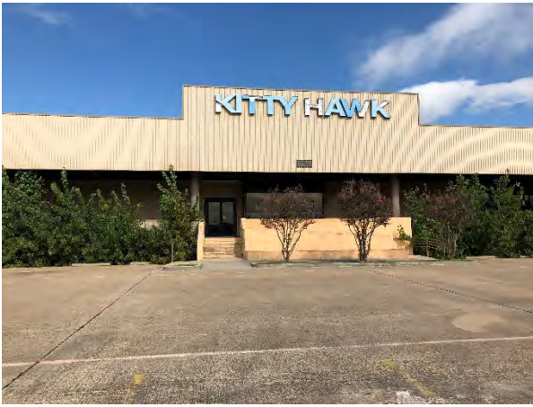
Photograph 1 – KHA Building, View to the North
