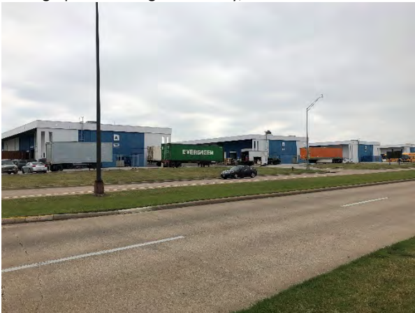
Photograph 23 – Building A, B, C, & D, View to Southeast
