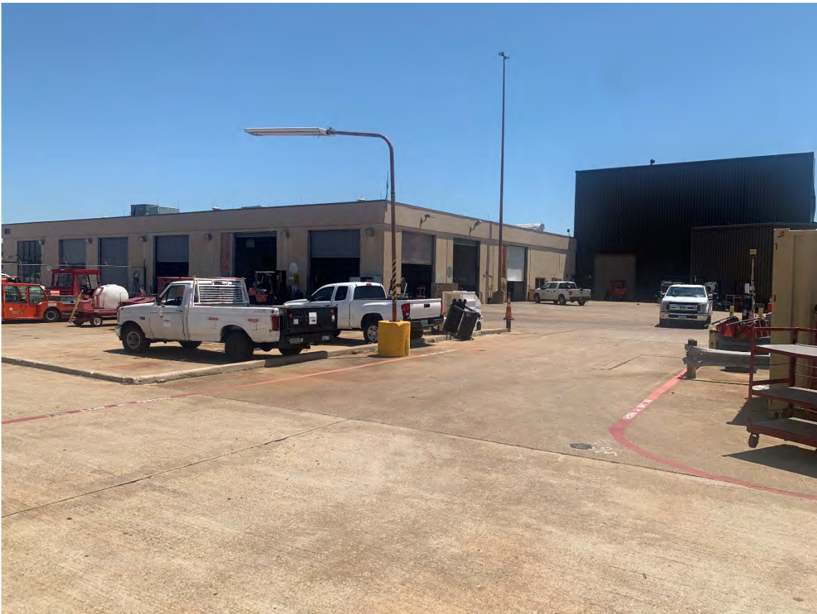
Photograph 18: American Airlines West Warehouse, south and west elevations, facing northeast.
