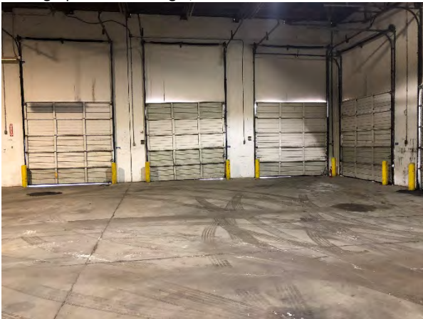
Photograph 55 – Building C, Interior
