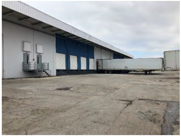
Photograph 26 – Building A, View to the East
