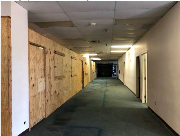
Photograph 15 – KHA Building, Interior
