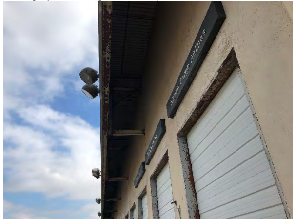
Photograph 6 - Evergreen Facility, View to the East
