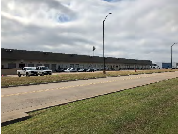
Photograph 3 - Evergreen Facility, View to the Southwest
