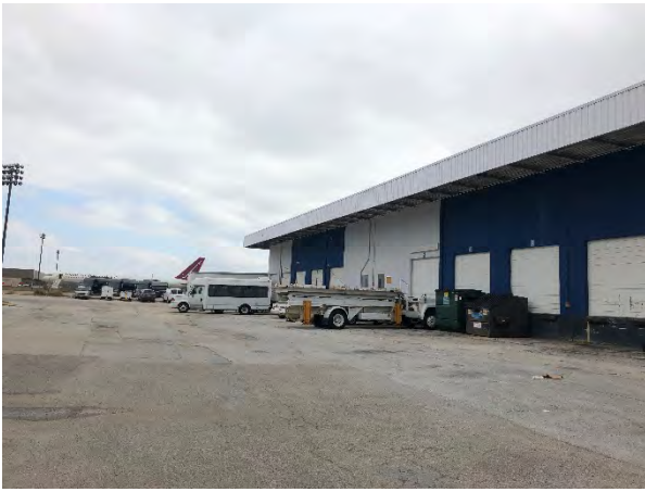
Photograph 49 – Building C, View to the Northeast
