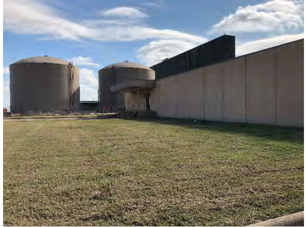
Photograph 12 – KHA Building, View to the Southeast
