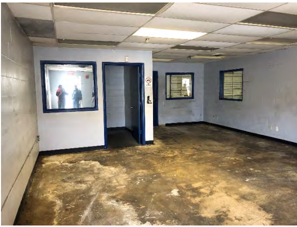
Photograph 57 – Building C, Interior
