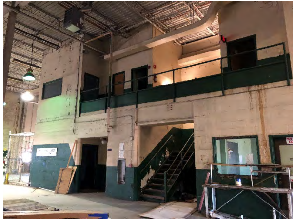
Photograph 18 – Evergreen Facility, Interior
