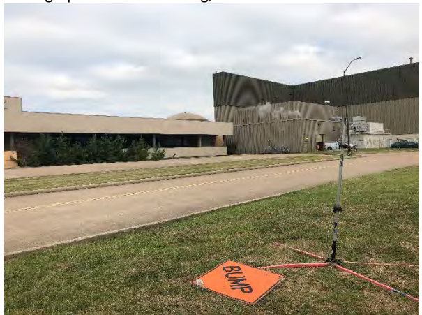
Photograph 22 – AA Hangar, View to the Northeast
