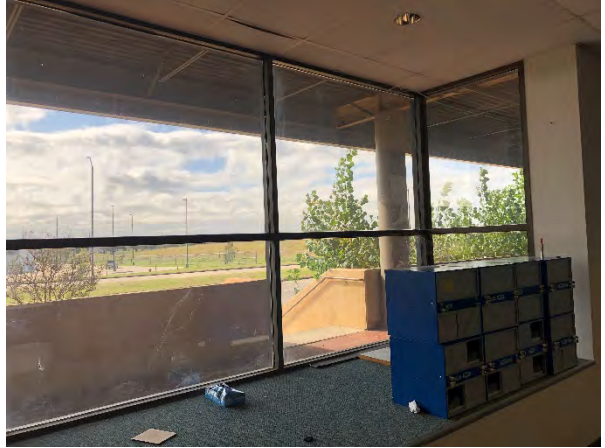
Photograph 20 – KHA Building, Interior
