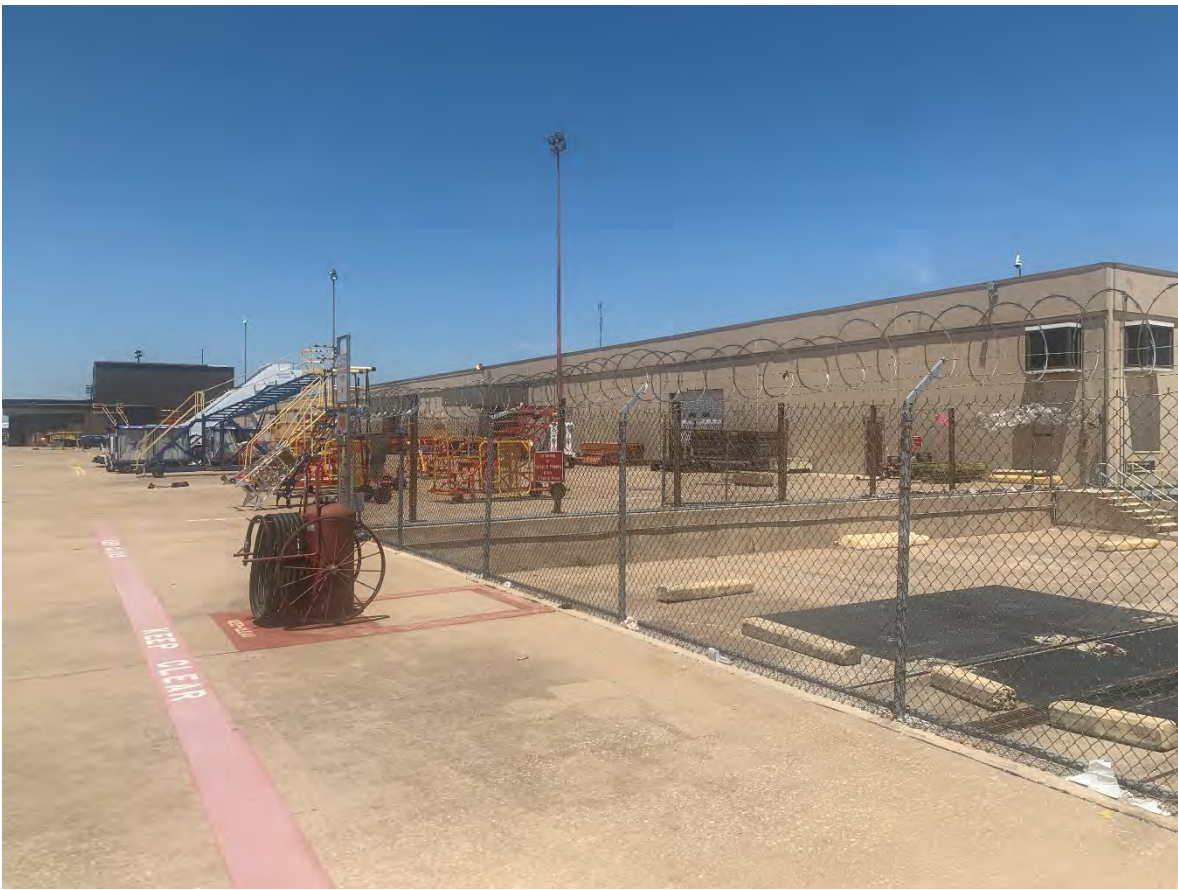
Photograph 13: American Airlines West Warehouse, south and east elevations, facing northwest.
