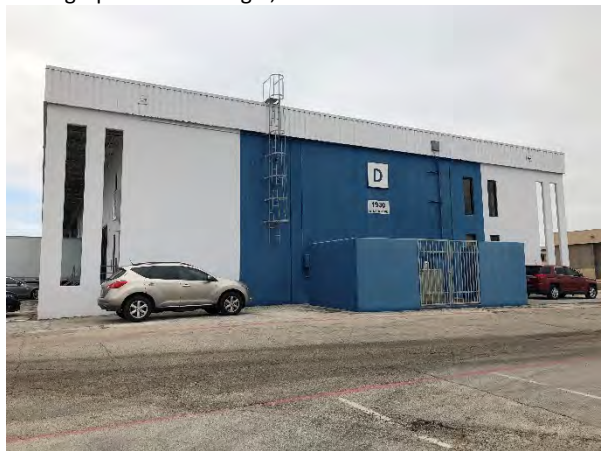
Photograph 62 – Building D, View to the East
