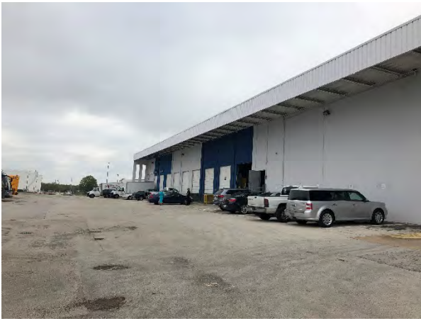
Photograph 33 – Building B, View to the Northwest
