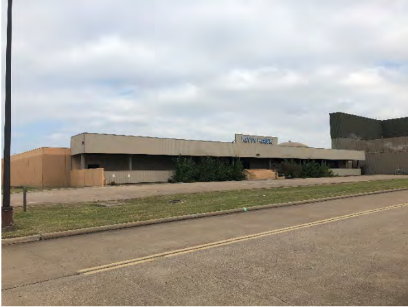
Photograph 3 – KHA Building, View to the Northeast
