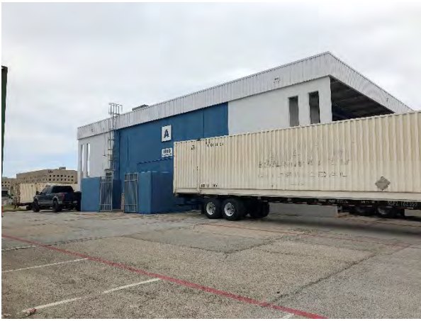
Photograph 25 – Building A, View to the Northeast
