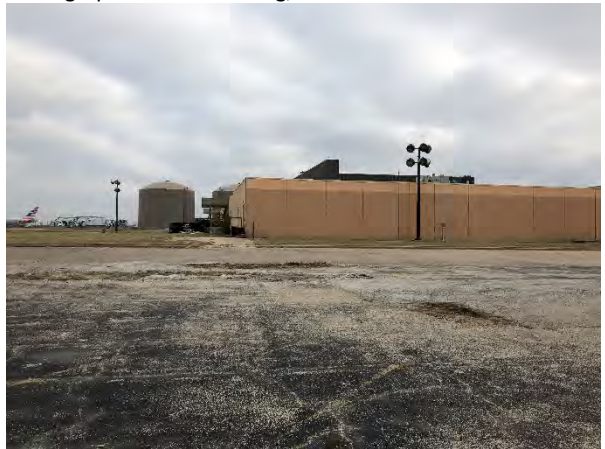
Photograph 8 – KHA Building, View to the East
