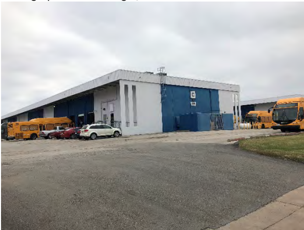
Photograph 47 – Building C, View to the Southeast
