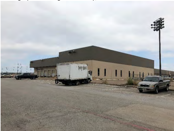
Photograph 7 - Evergreen Facility, View to the Northwest
