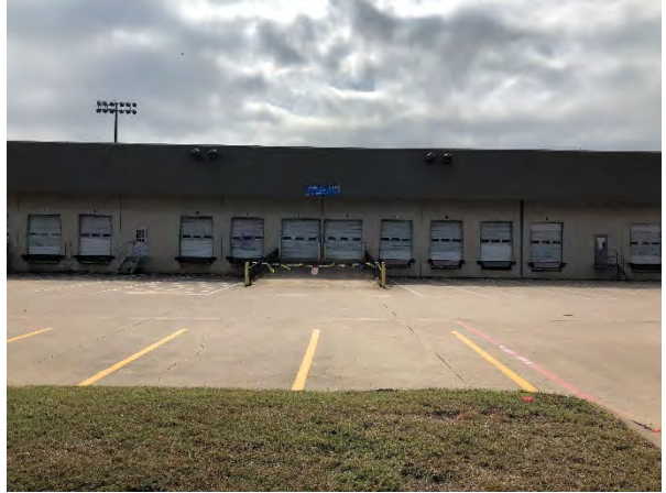
Photograph 4 - Evergreen Facility, View to the South
