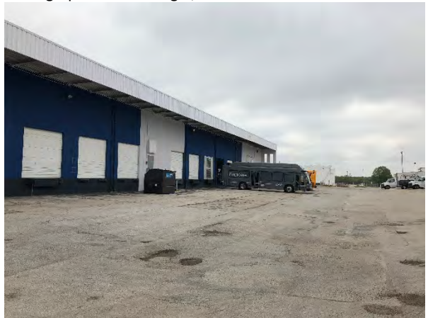
Photograph 48 – Building C, View to the Southwest
