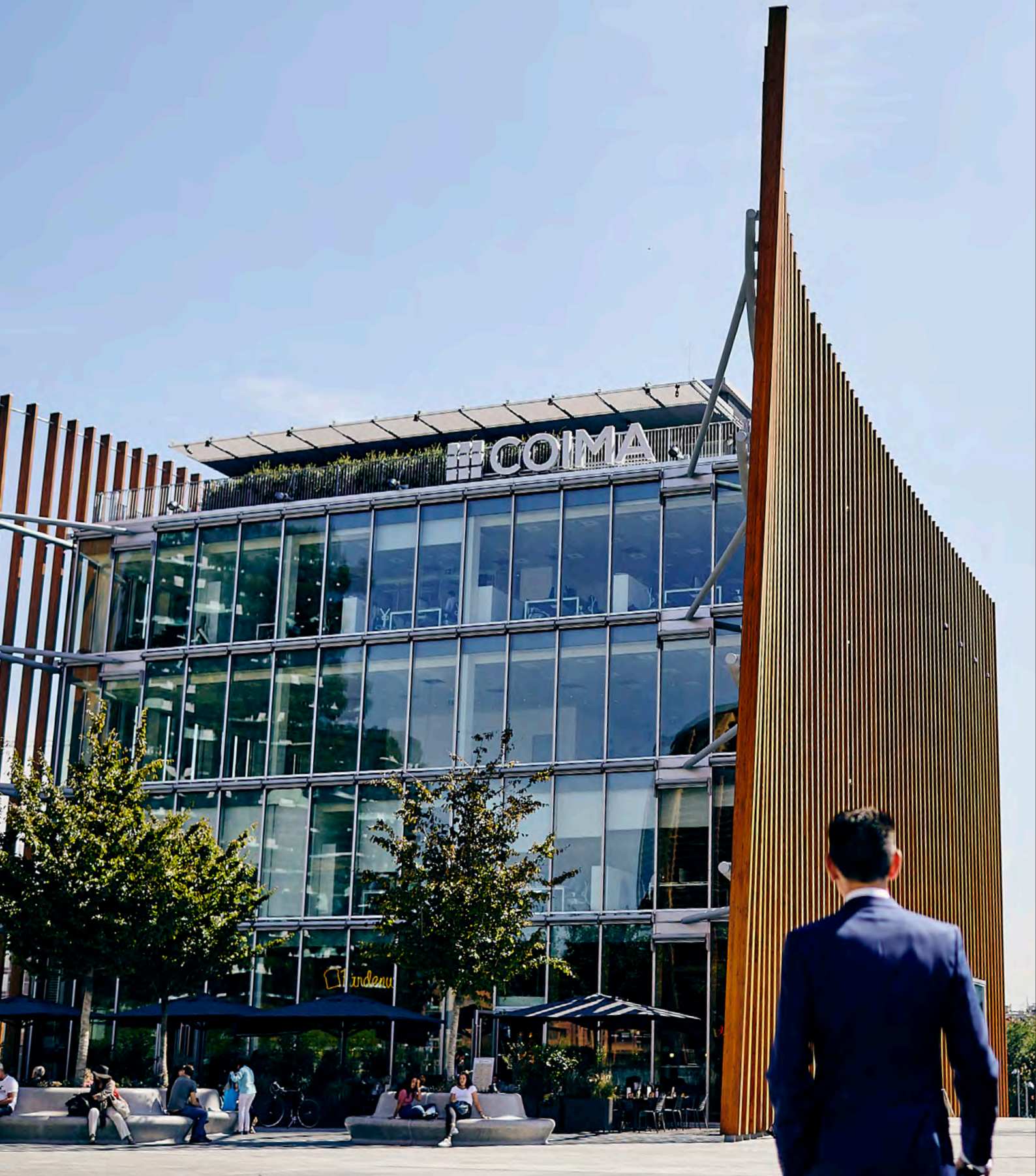
Milano, COIMA Headquarters
