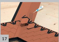
In the valley, lay a roll of roof membrane of the same colour of a width of 1 metre. The roll should be stapled on both sides, with approx. 6 cm between the nails. Mark the valley width approx. 15 cm on each side of the roof and apply 3 lines of Icopal Roof Glue.
