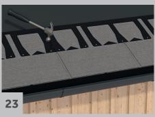
The shingle should be stapled to the substrate in the adhesive field as shown in the figure. During installation, check regularly that the shingle rows are straight and parallel with the eaves. The shingle plates must never be displaced upwards on the roof to align with the horizontal, as the material will not be sufficient.
