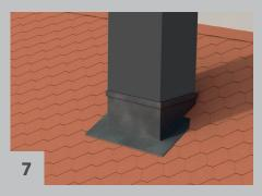
The shingle should be laid right up to the side of the fitting.
