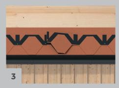
The first row of shingles should be laid so that the tongues are flush with the lower edge of the base plate and cover the adhesive fields. The guide track will give the correct internal height of the shingle sheets.
