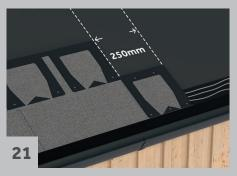
Mark two parallel lines with chalk approximately in the middle of the roof. The distance should be equal to the width of half of the tongue of the shingle. Start laying one row of the shingles and continue towards the sides. The next row should start by the other row.
