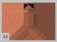
At the end of the ridge plates on a hip roof, a ridge plate should be split into two pieces. They should cover the Y-shaped surface and be nailed down. Nearly all of the ridge plates should be laid so as to cover the "split". The last one should be glued into place.
