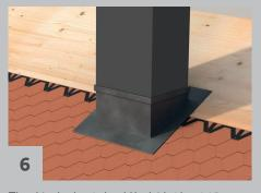
The shingle sheet should be laid at least 15 cm past the front edge of the pipe, so that the fitting will cover the shingle row at the front edge of the chimney. Apply 3 lines of Icopal Roof Glue to the remaining shingle under the flange of the fitting flange. Fit the chimney fitting.
