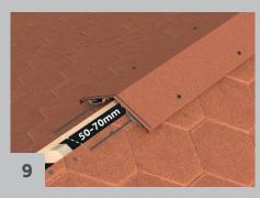
The gap in the ridge must be covered approx. 25 cm from the outer wall and 40 cm on the side in the case of a T-ridge.
