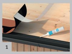
The combined eave/ridge plate should be laid parallel along the eaves. Cord should be used to maintain the alignment.
