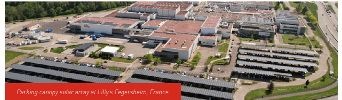
Parking canopy solar array at Lilly's Fegersheim, France
