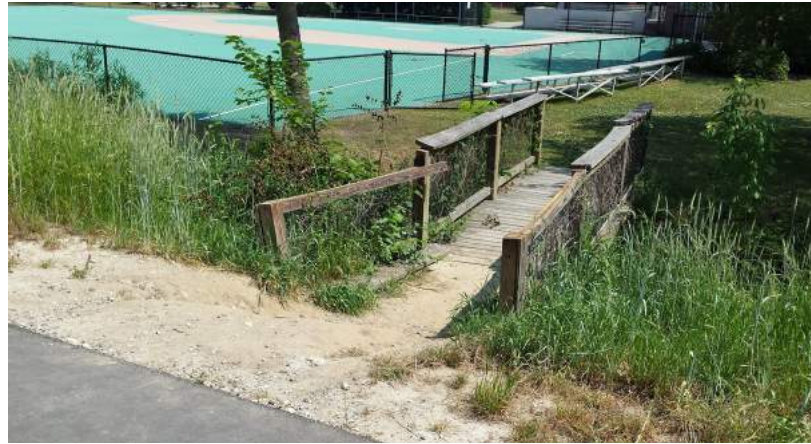
Forest Park bridge connection to Bikeway, poor condition + grading issues.
