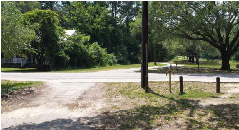
Bikeway crossing at White Oak Drive. Bikeway crossings typically lack definition, signage, and street markings.
