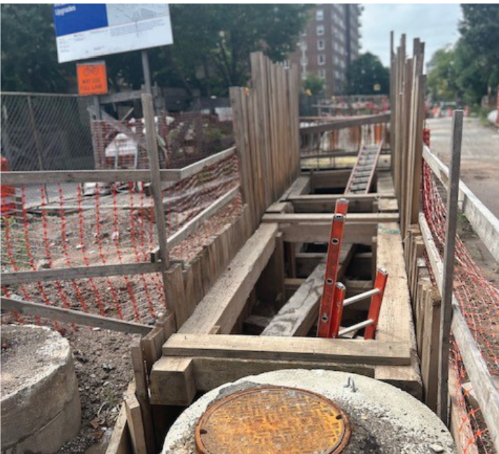
Photo 1: Installation of new proposed 24-inch reinforced concrete pipe combined sewer at Vanderbilt Ave; Photo 2: Removal of storage area and fencing by 250 Park Pl.;
