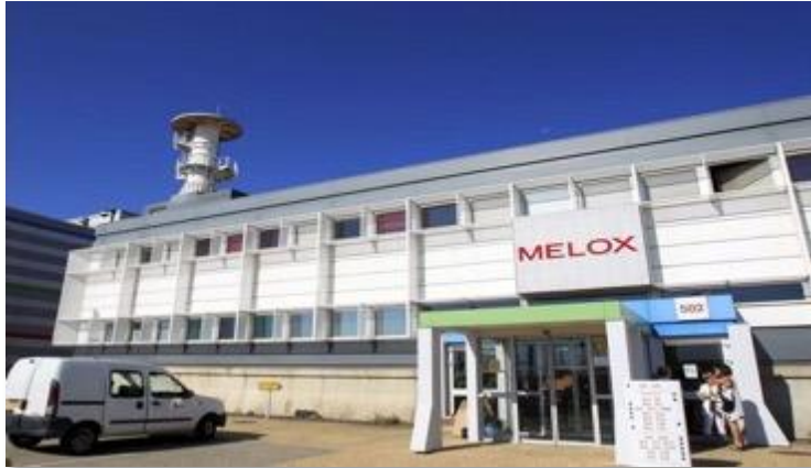
MELOX, currently the world's only commercial MOX fuel production facility, was built in 1995 in France
