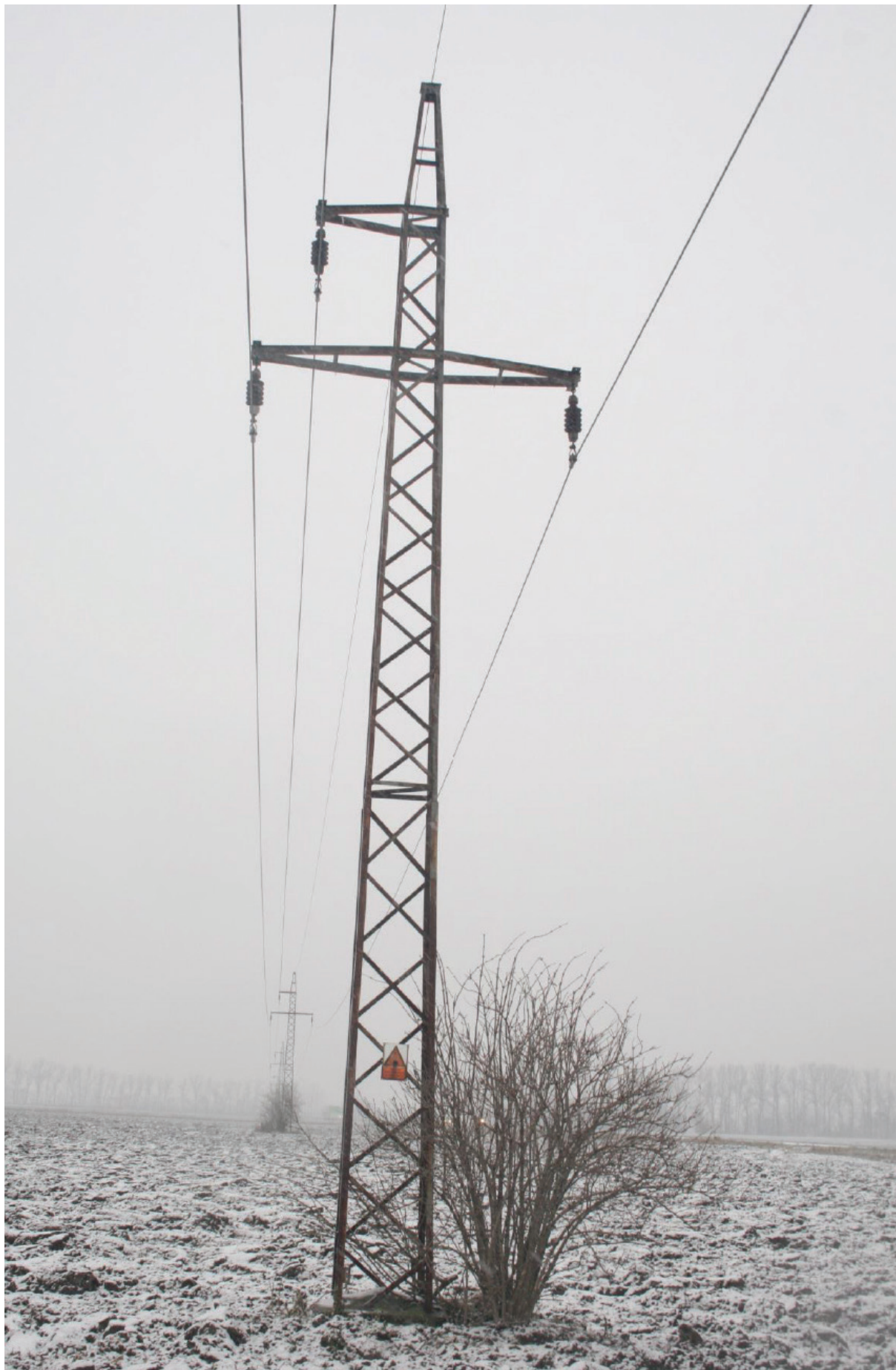
Fig. 12: Low risk: Electric pole with hanging insulators. © Raptor Protection of Slovakia
