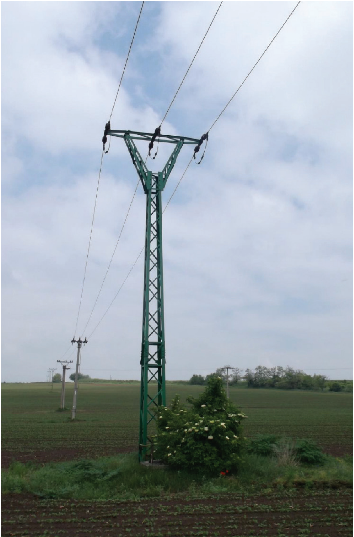
Fig. 9: Medium risk: Electric pole with hanging exposed jumper wires below the console. © Raptor Protection of Slovakia
