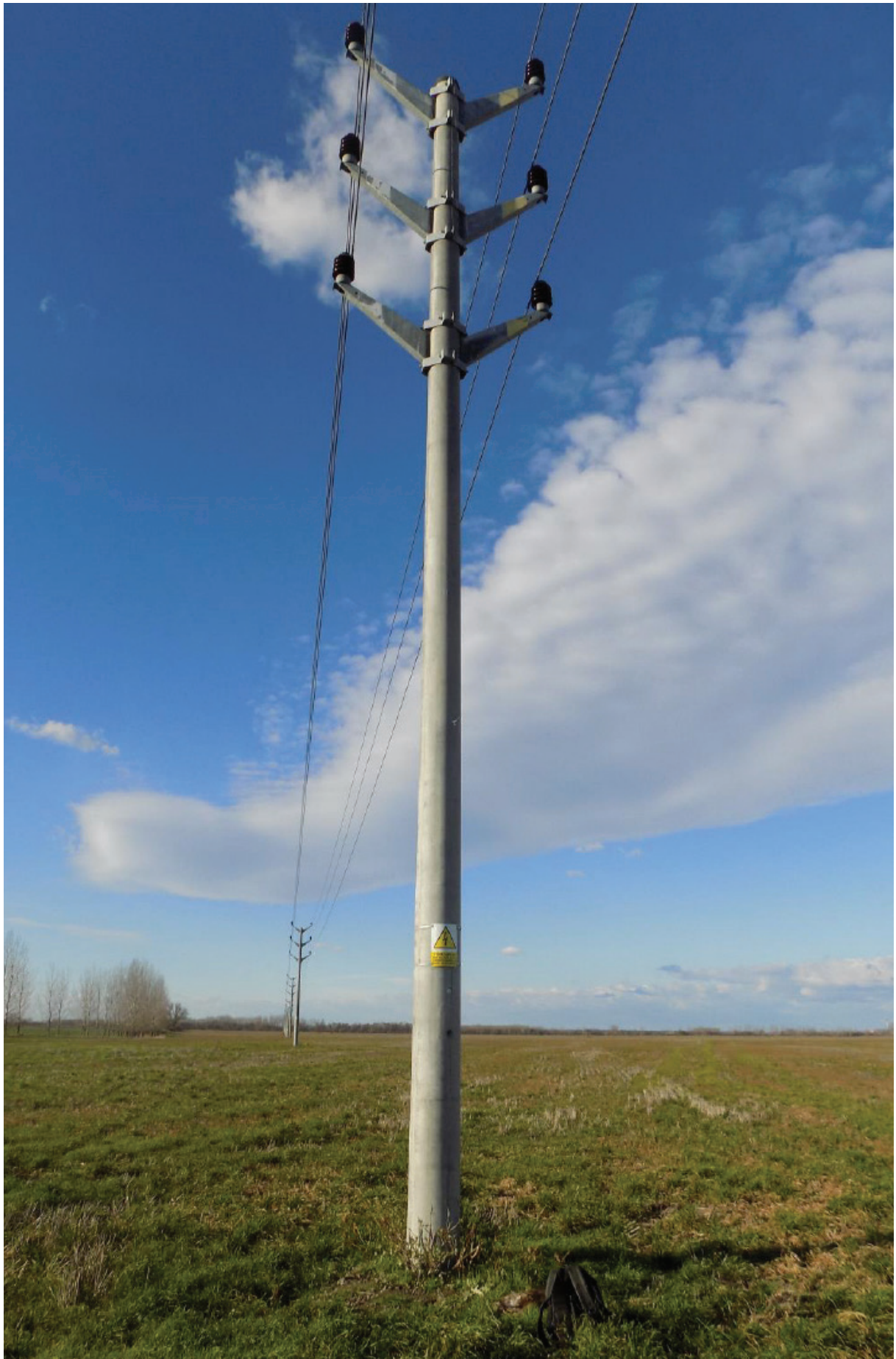
Fig. 13: Low risk: Double circuit electric pole with 45° angle of the arms. © Raptor Protection of Slovakia
