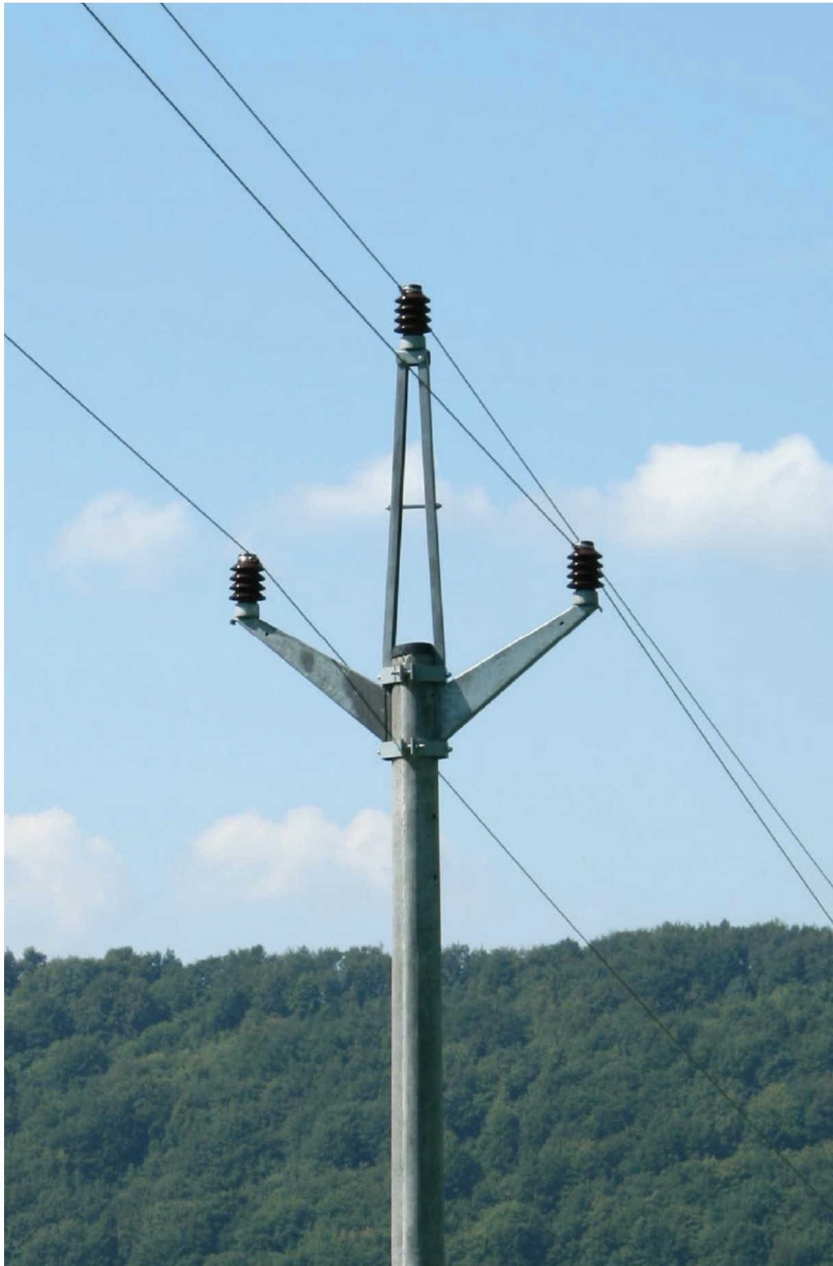
Fig. 10: Low risk: Electric pole with 45° angle of the arms. © Raptor Protection of Slovakia
