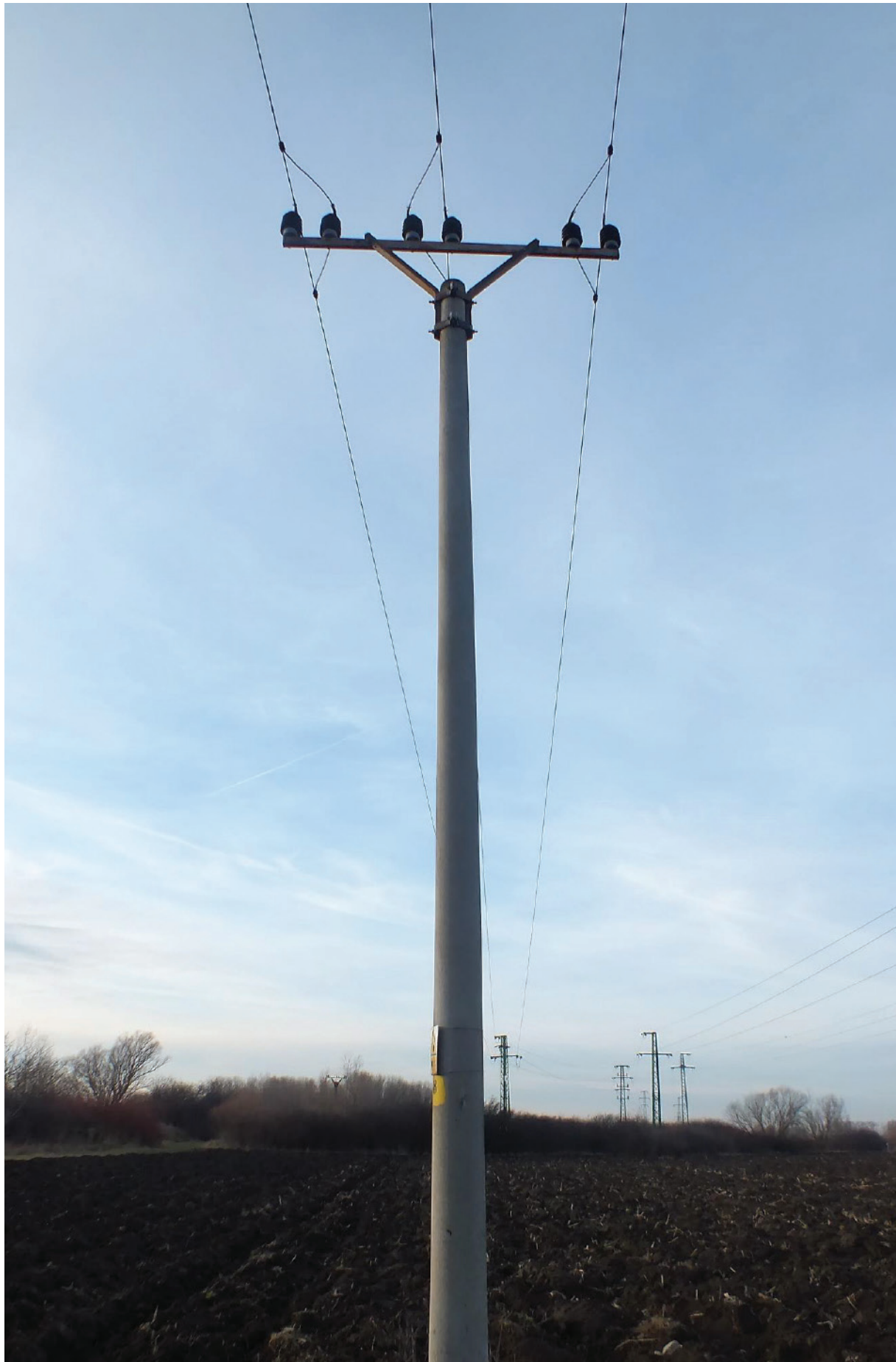
Fig. 6: Medium risk: Electric pole with a pair of support insulators in vertical position on console. © Raptor Protection of Slovakia
