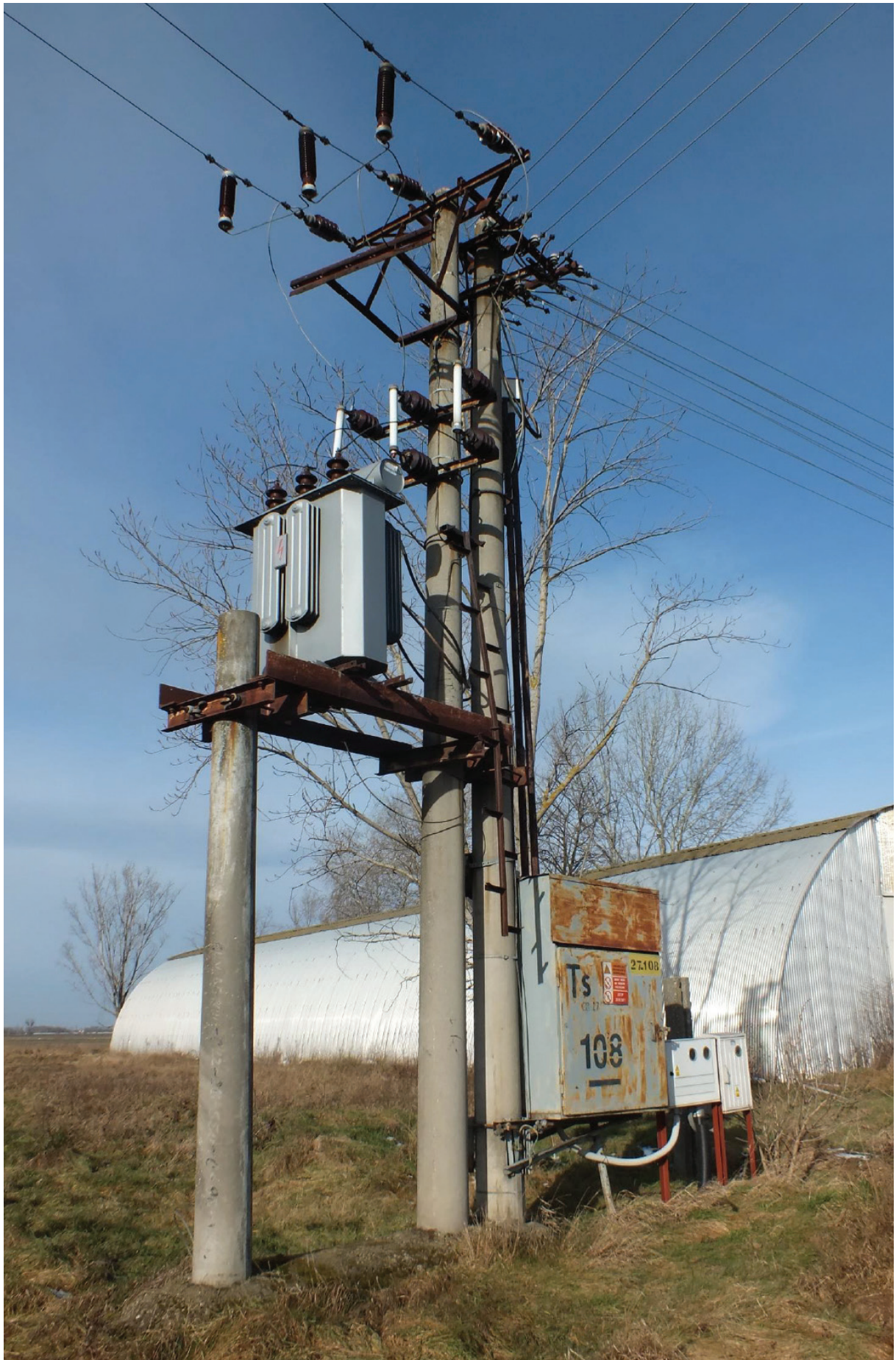
Fig. 7: Medium risk: Electric pole transformer with a combination of exposed jumper wires locations. © Raptor Protection of Slovakia
