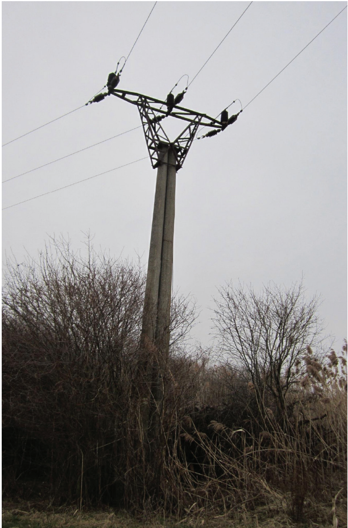
Fig. 4: High risk: Electric pole with three exposed jumper wires above the console. © Raptor Protection of Slovakia
