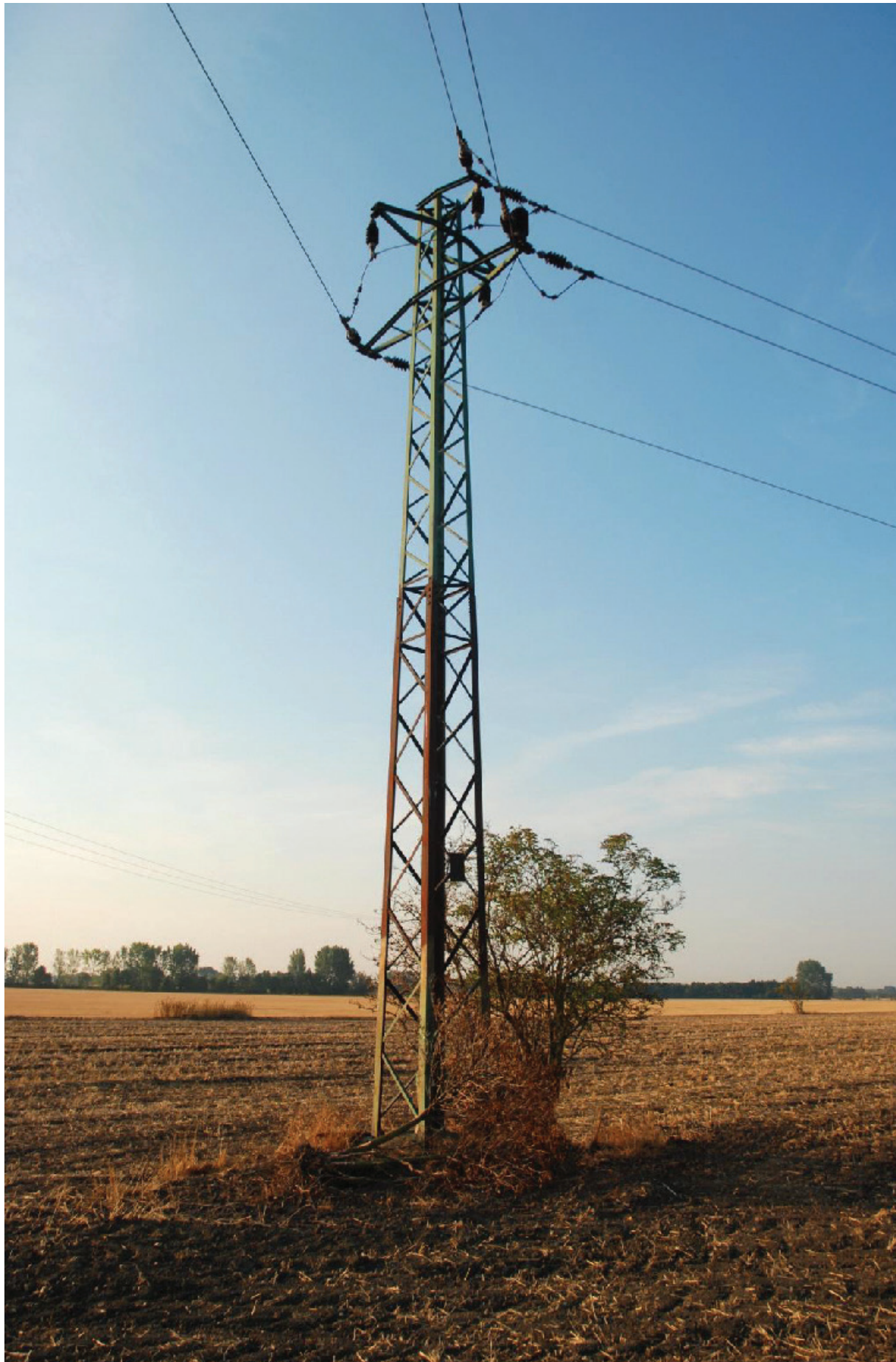
Fig. 2: High risk: Corner pylon with a combination of support insulators and exposed jumper wire locations. © Raptor Protection of Slovakia
