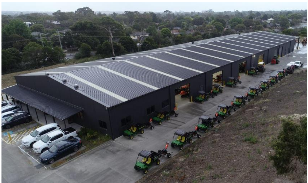
Peninsula Kingswood Country Golf Club Maintenance Facility Source: Turfmate
