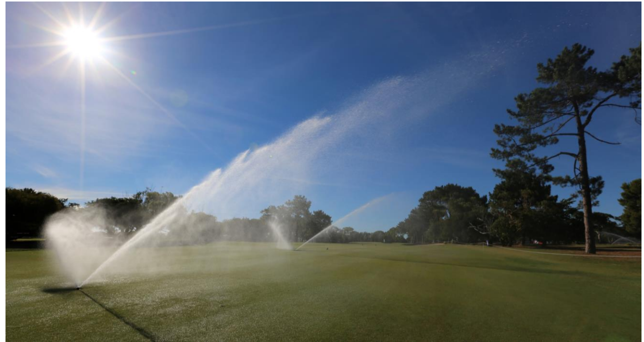
Image of a fairway automatic irrigation system
