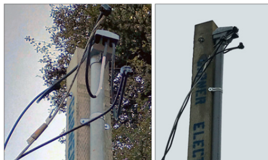
Figure 17. Typical Temporary Weatherhead Installation (Front view on left, side view on right)
