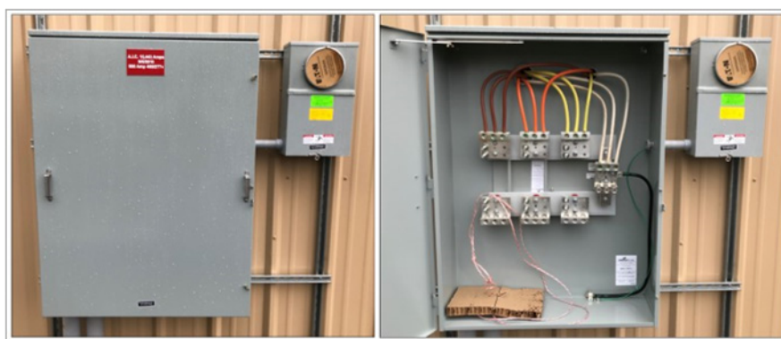
Figure 94. Typical Horizontal Current Transformer Metering Installation
