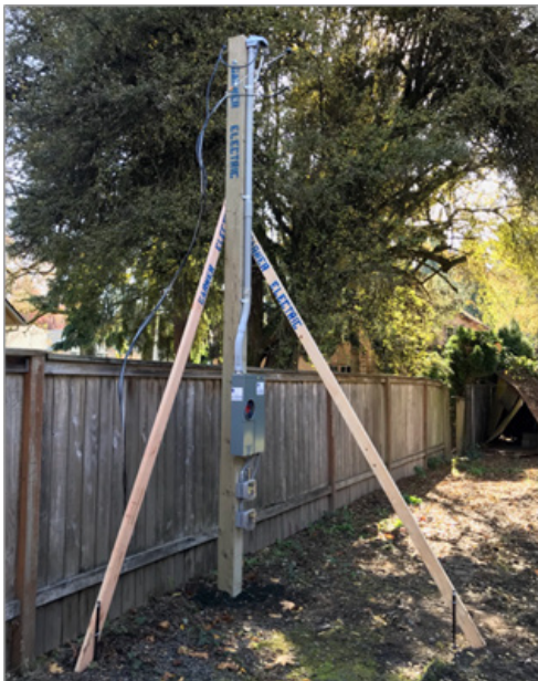
Figure 15. Typical Overhead-Service Post
