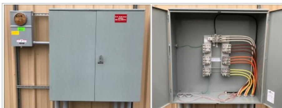
Figure 95. Typical Vertical Current Transformer Metering Installation
