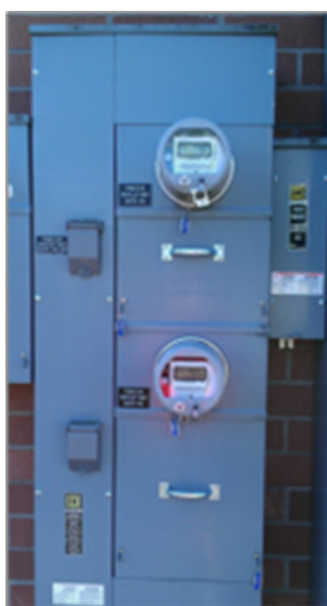
Figure 90. Typical Double-Stacked Module Meter Sockets
