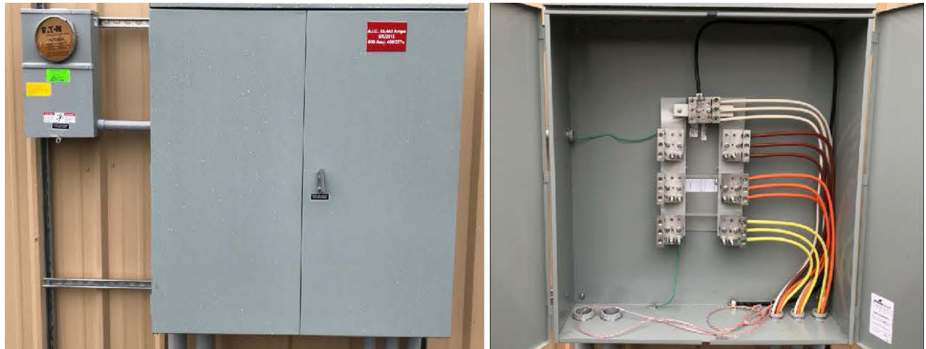
Figure 84. Typical Vertical Current Transformer Metering Installation
