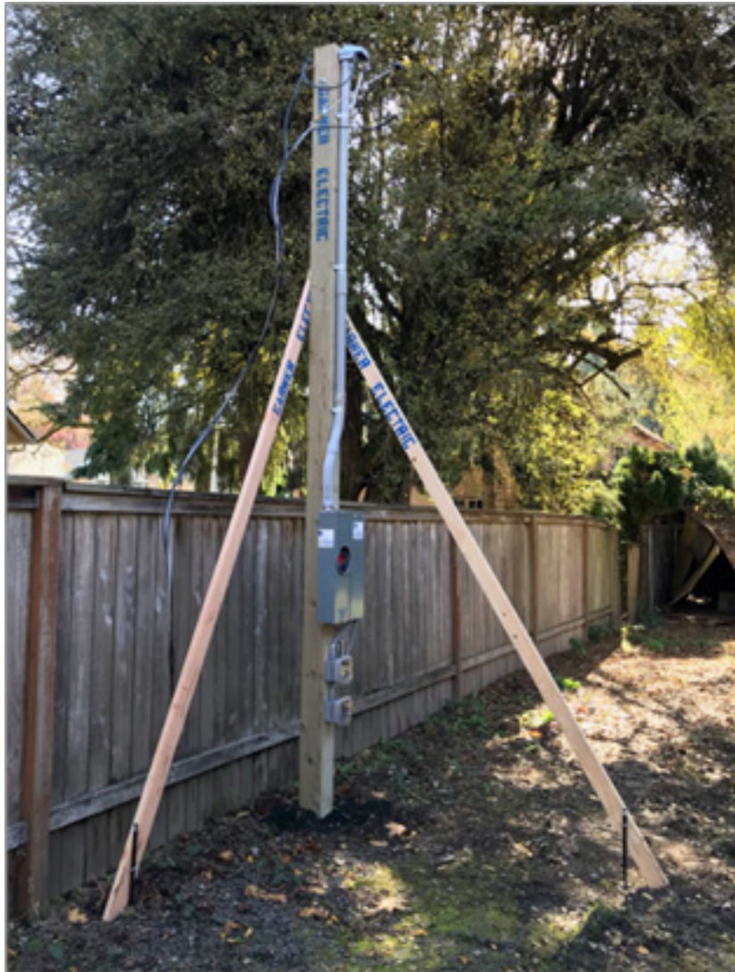
Figure 10. Typical Overhead Service Post
