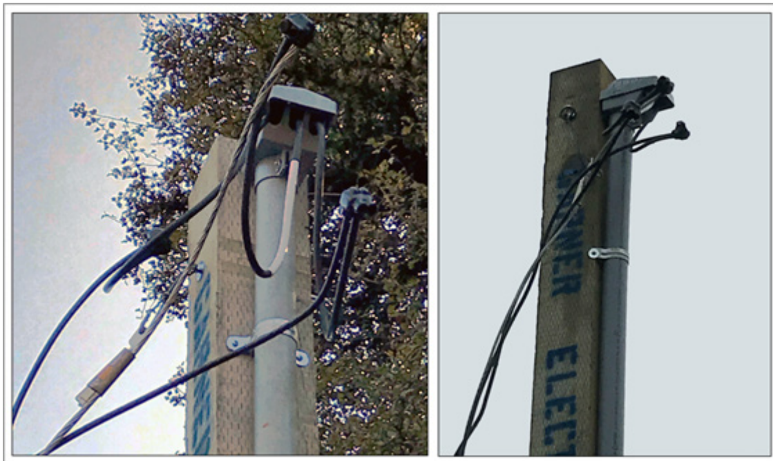
Figure 12. Typical Temporary Weatherhead Installation (Front view on left, side view on right)
