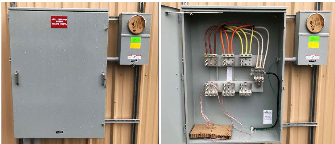
Figure 83. Typical Horizontal Current Transformer Metering Installation
