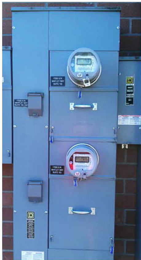
Figure 79. Typical Double-Stacked Module Meter Sockets
