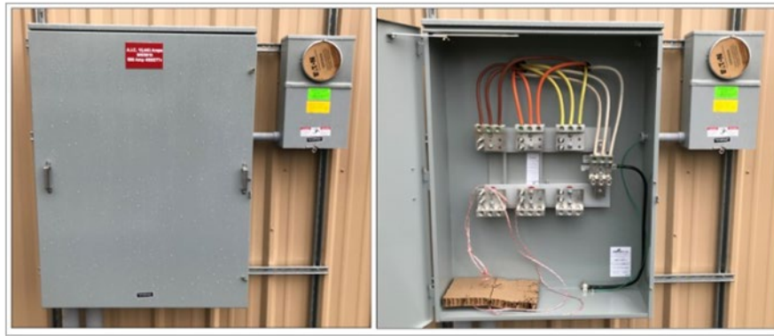
Figure 93. Typical Horizontal Current Transformer Metering Installation
