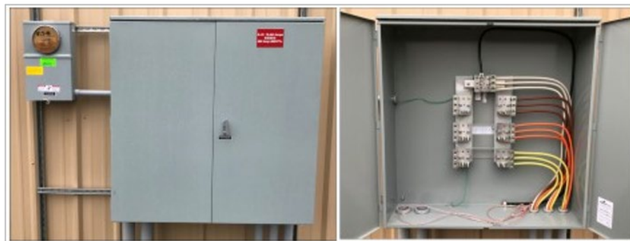
Figure 94. Typical Vertical Current Transformer Metering Installation
