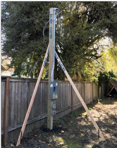
Figure 15. Typical Overhead-Service Post
