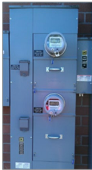
Figure 89. Typical Double-Stacked Module Meter Sockets
