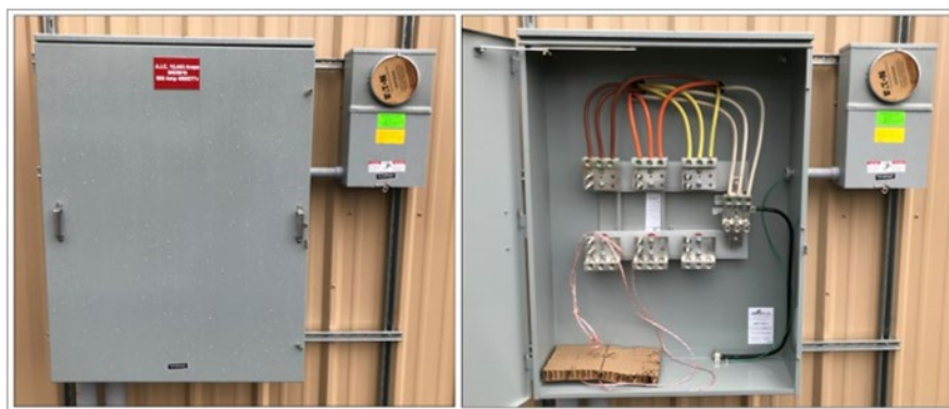
Figure 93. Typical Horizontal Current Transformer Metering Installation
