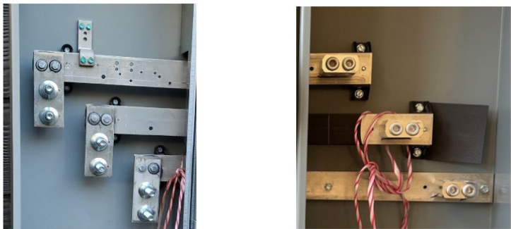
Figure 71. Examples of Service Terminating Arrangements for Two- and Three Multi-meter Packs
