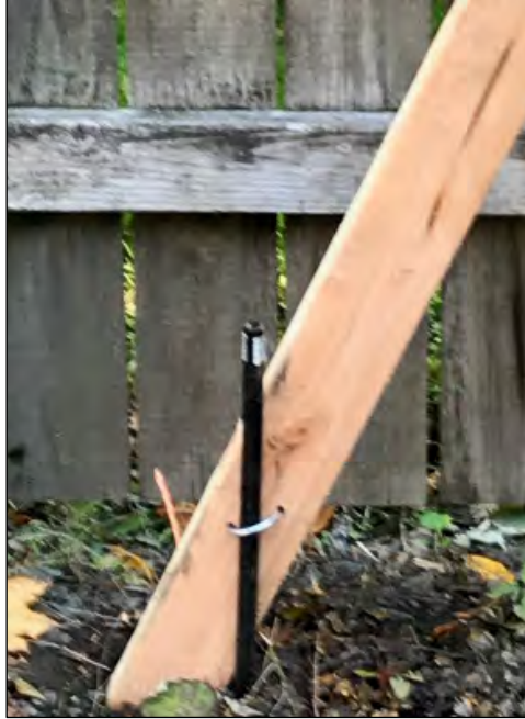
Figure 9: Typical Steel Stake and Brace Installation
