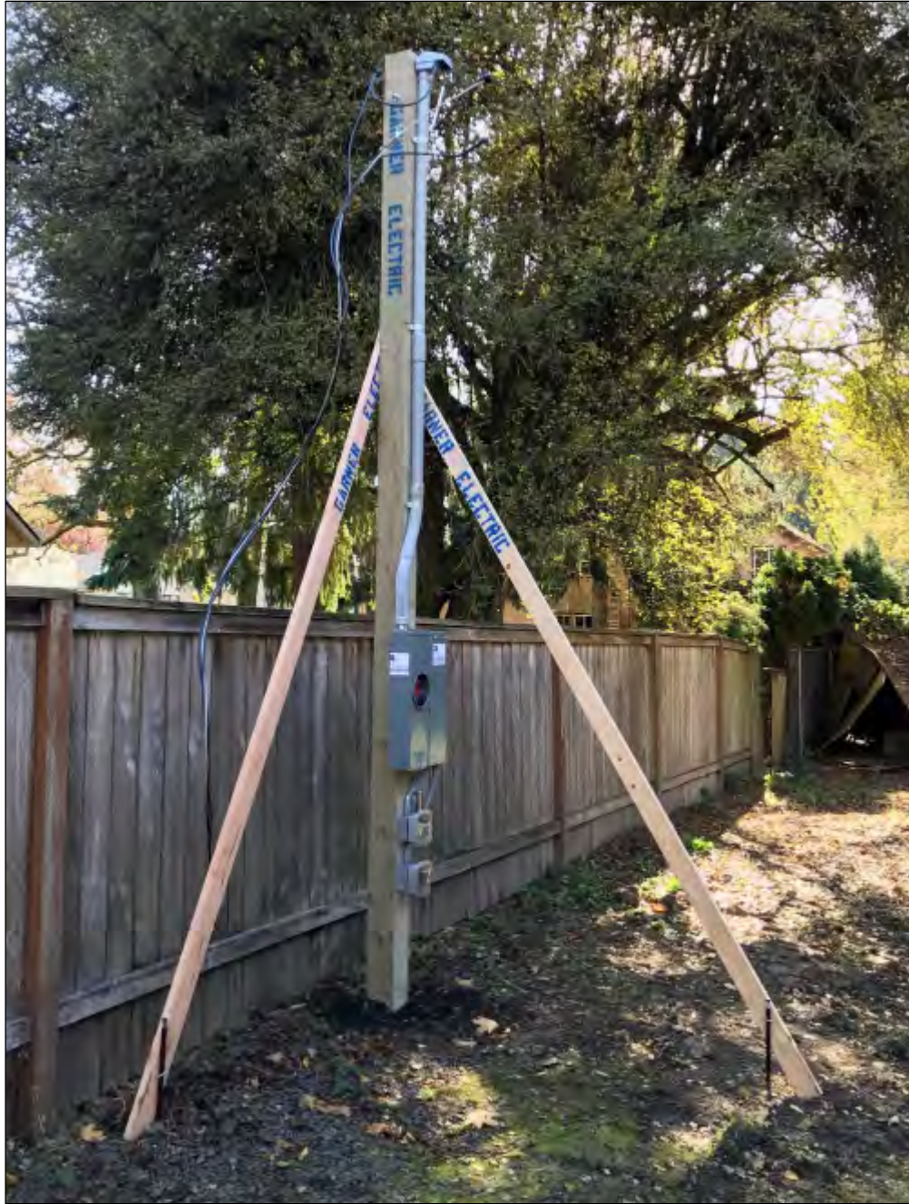
Figure 5: Typical Overhead Service Post
