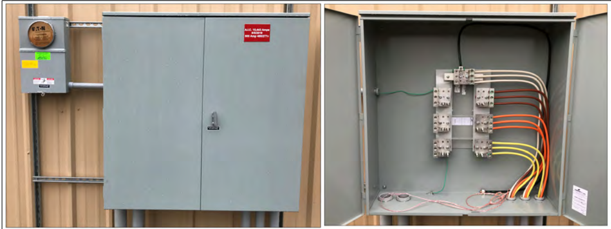
Figure 76: Typical Vertical Current Transformer Metering Installation
