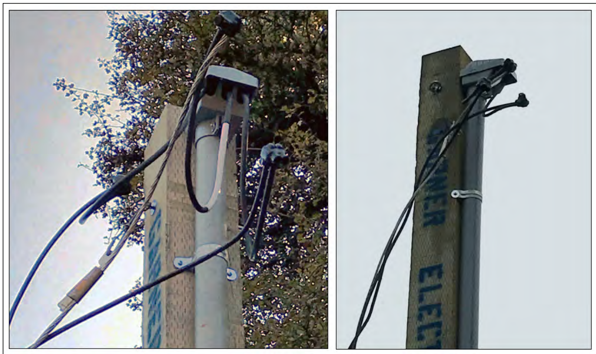
Figure 7: Typical Temporary Weatherhead Installation (Front view on left, side view on right)
