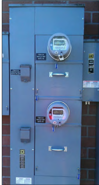
Figure 69: Typical Double-Stacked Module Meter Sockets
