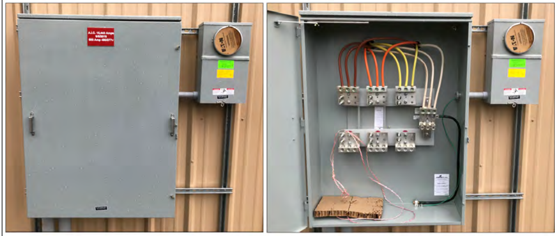
Figure 74: Typical Horizontal Current Transformer Metering Installation
