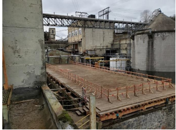
Mill J foundation after demolition
