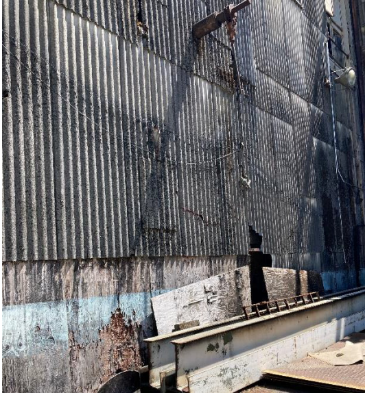
Transite (asbestos) siding
