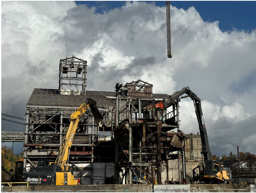
Sawmill demolition begins
