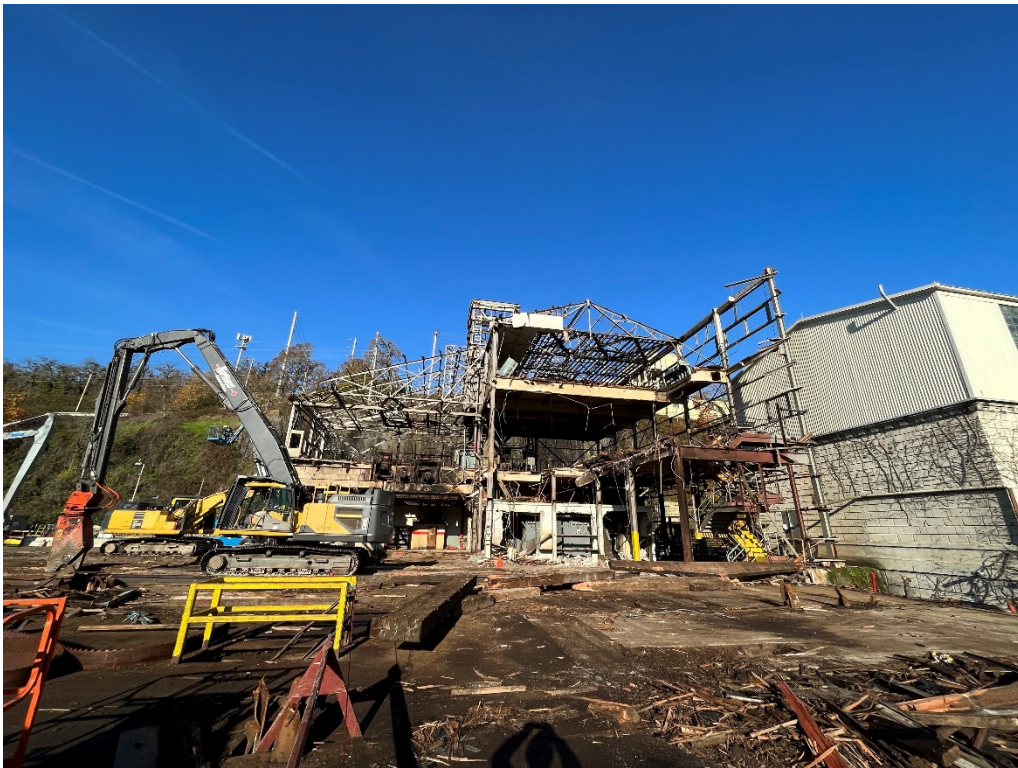
Remainder of Sawmill is dismantled
