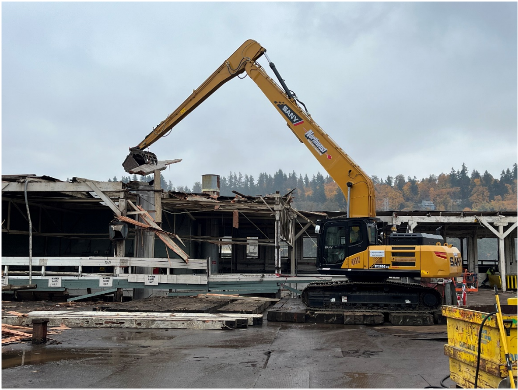
Removing the roof of Grinder Room #2
