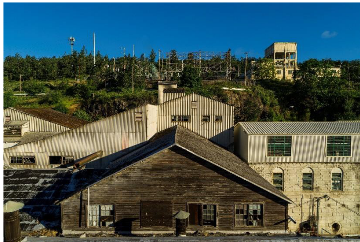
Rooflines from the East
