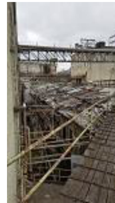
Mill J roof
