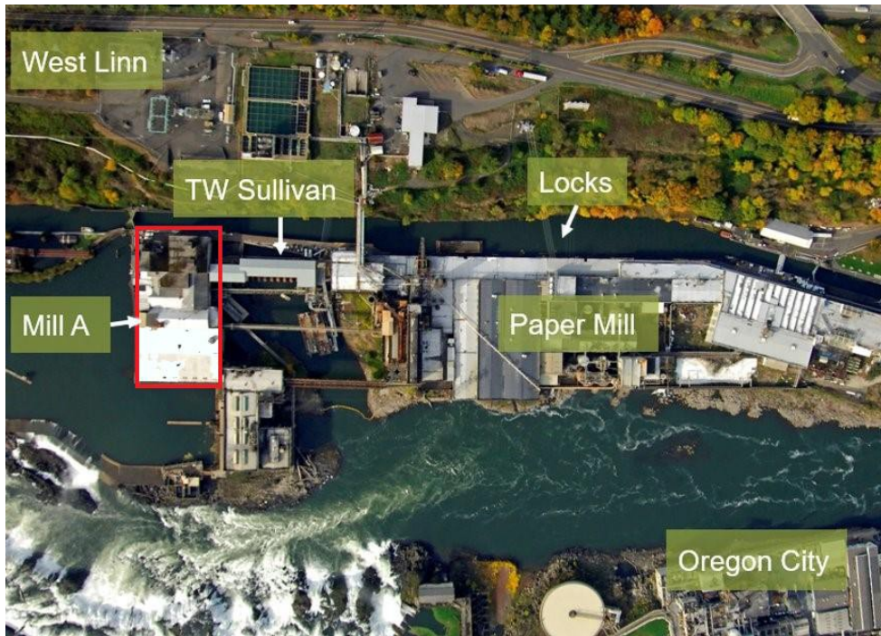
An overview of Mill A and Moore Island
