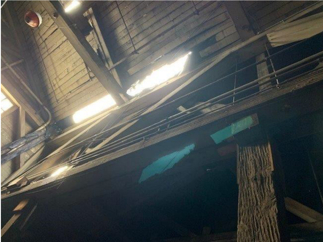
Decayed roofing
