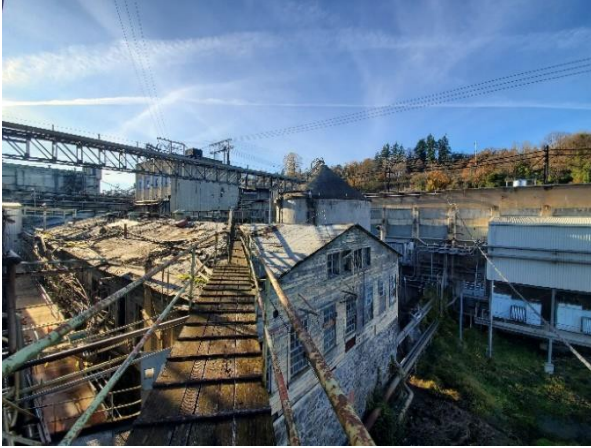
Mill J before demolition
