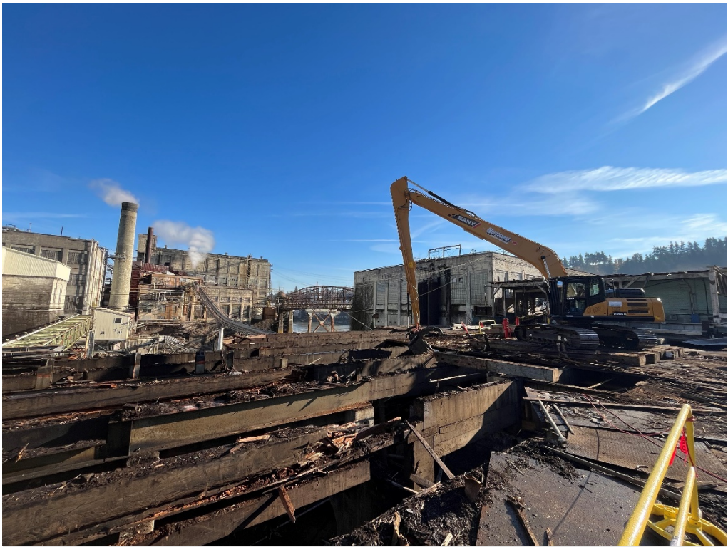
Main decking in the Central Area is removed
