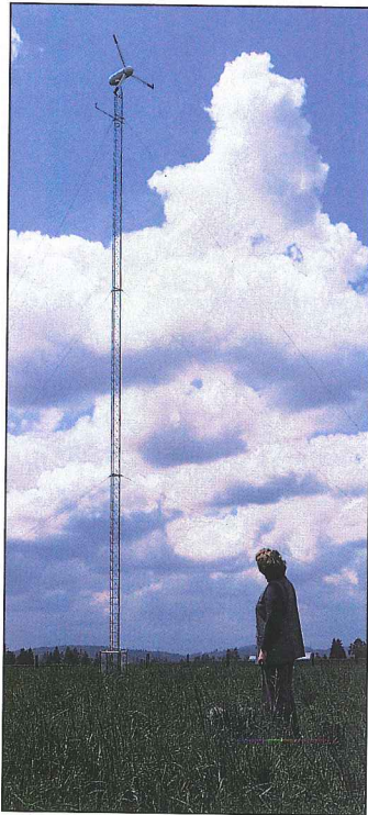
A windmill generates electricity on a Gresham farm.
