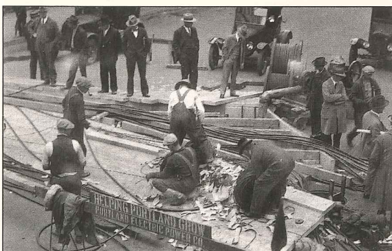
Installing Portland's first traffic lights, 1938.
