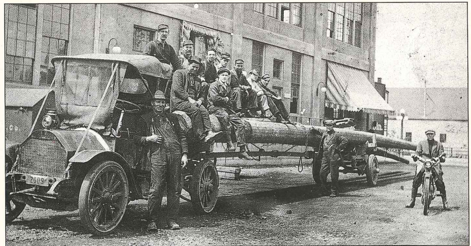
By 1913, line crews used a three-speed pole truck.
