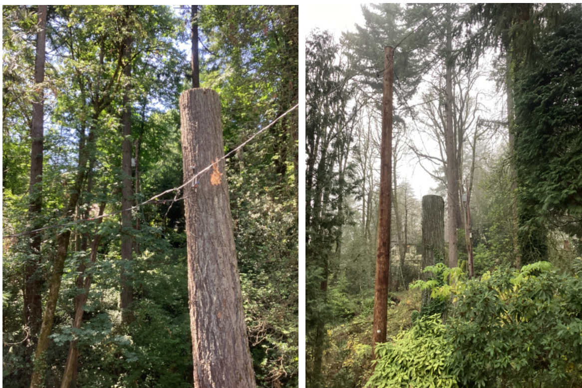
Figure 7-7: Service Conductor Attached to Tree (left) and Correction (right)
