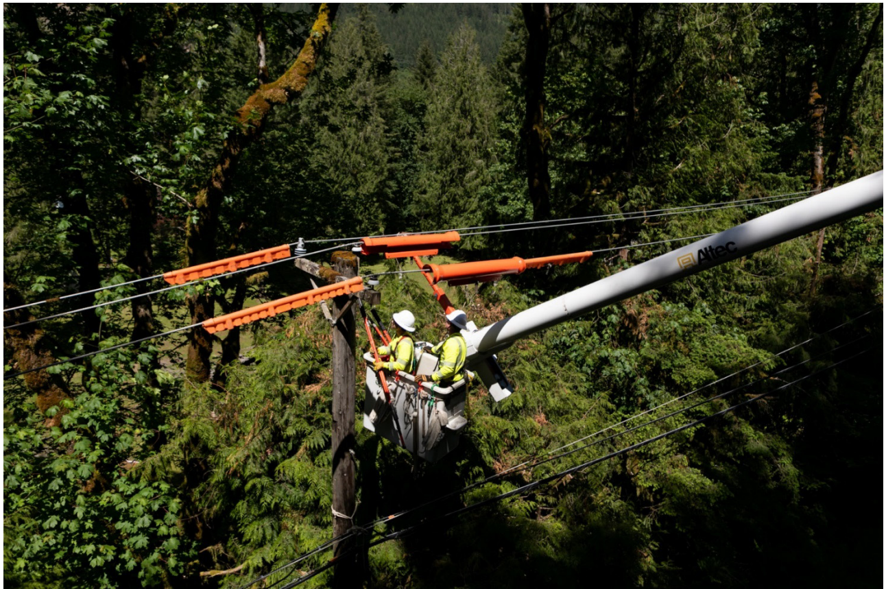
Figure 5-6: Crews Conduct Cross-Arm Replacement
