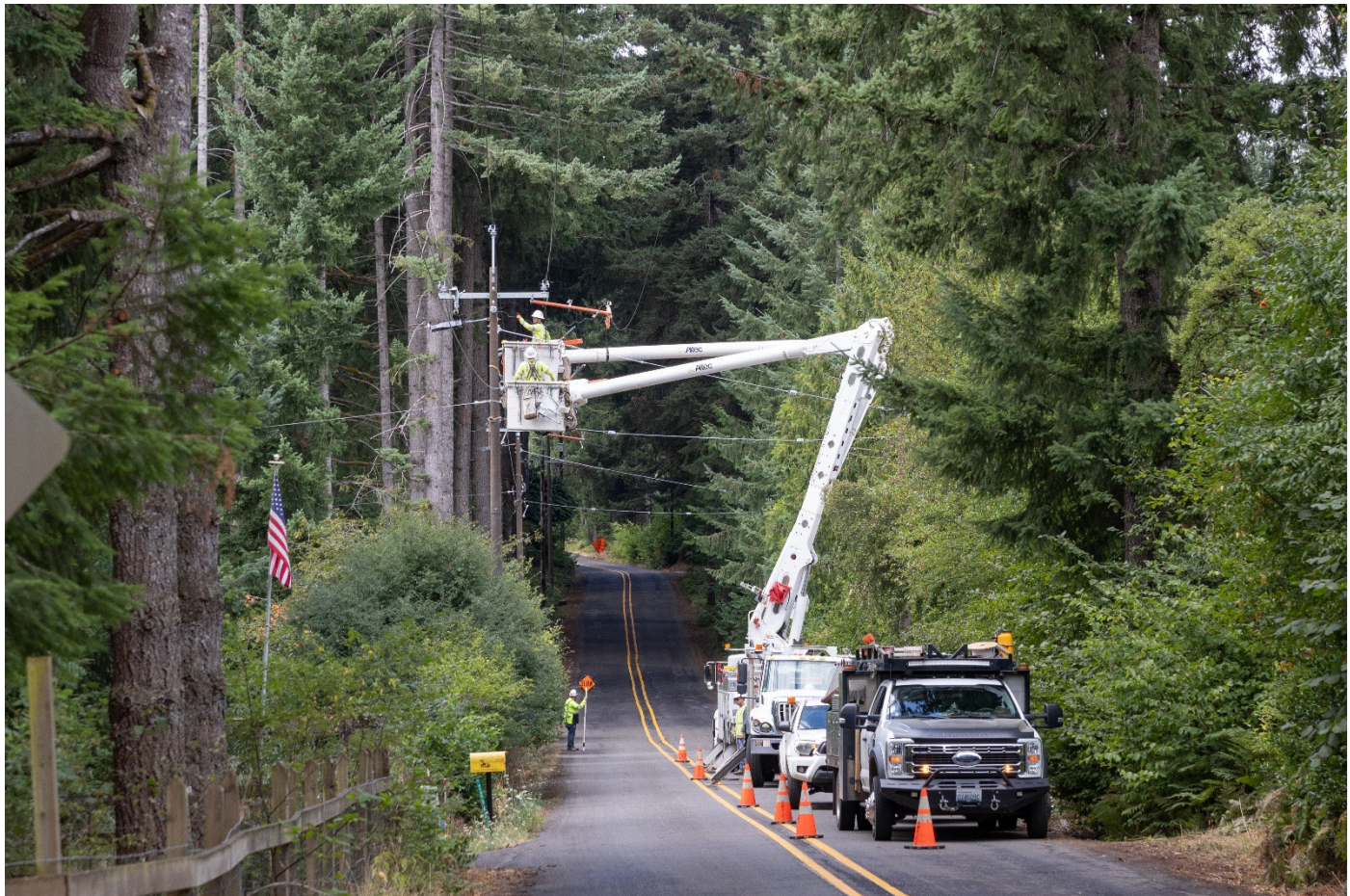
Figure 6-3: Covered Conductor installation on Leland-Carus
