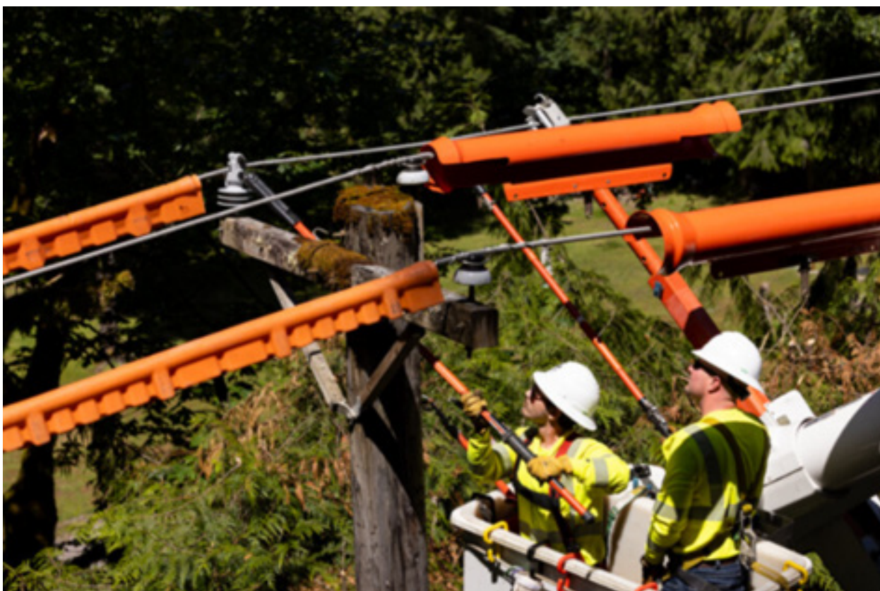
Figure 7-6: Ignition Prevention Crew Replacing Insulator
