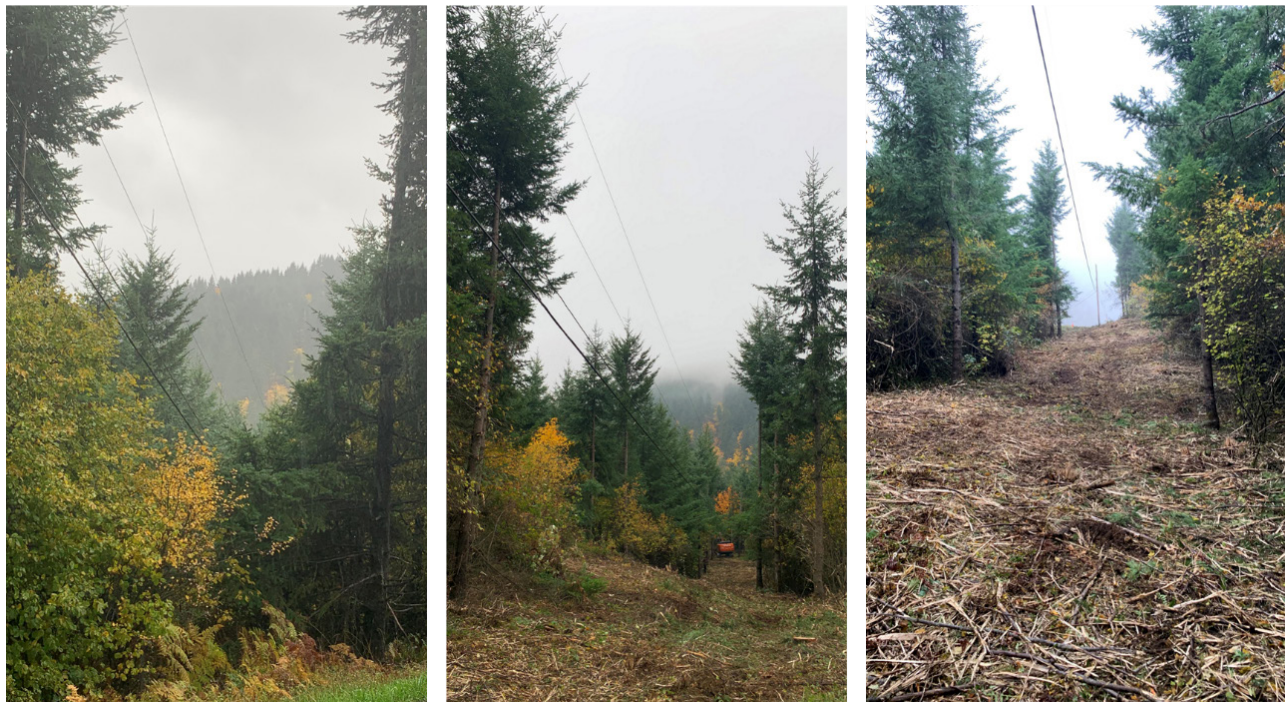
Figure 8-8: Heavily Vegetated Corridor Mowing Pre- and Post-Mitigation
