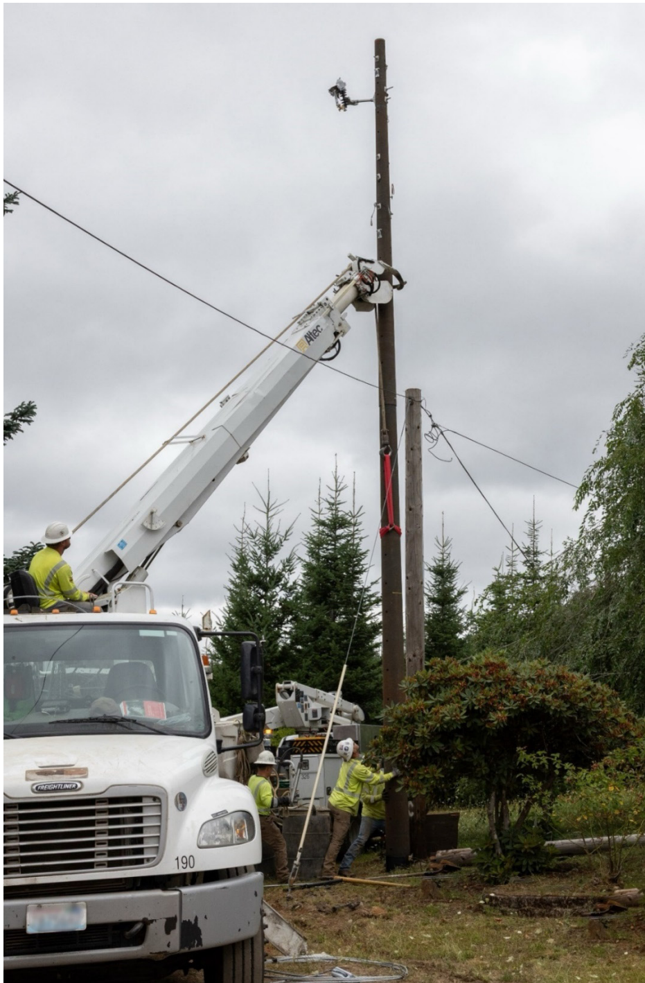
Figure 6-5: Distribution pole replacement with Ductile Iron pole
