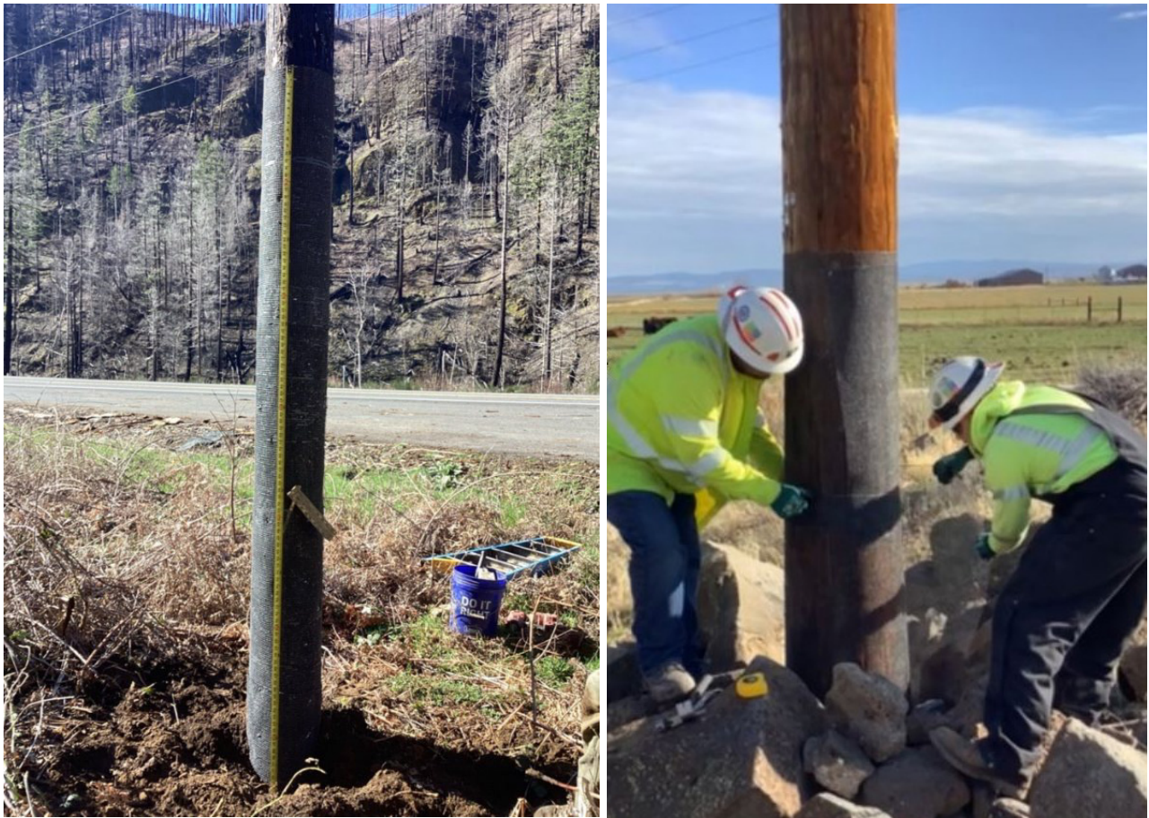
Figure 6-4: Fire Mesh Pole Wrap Installation
