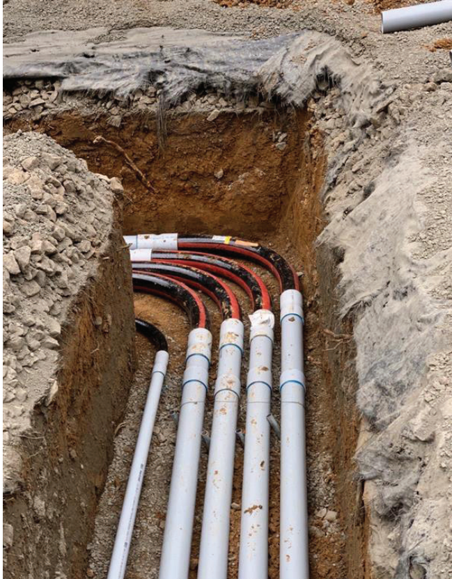
Figure 12. Conduit Spacers Required for Multiple Conduit Installation
