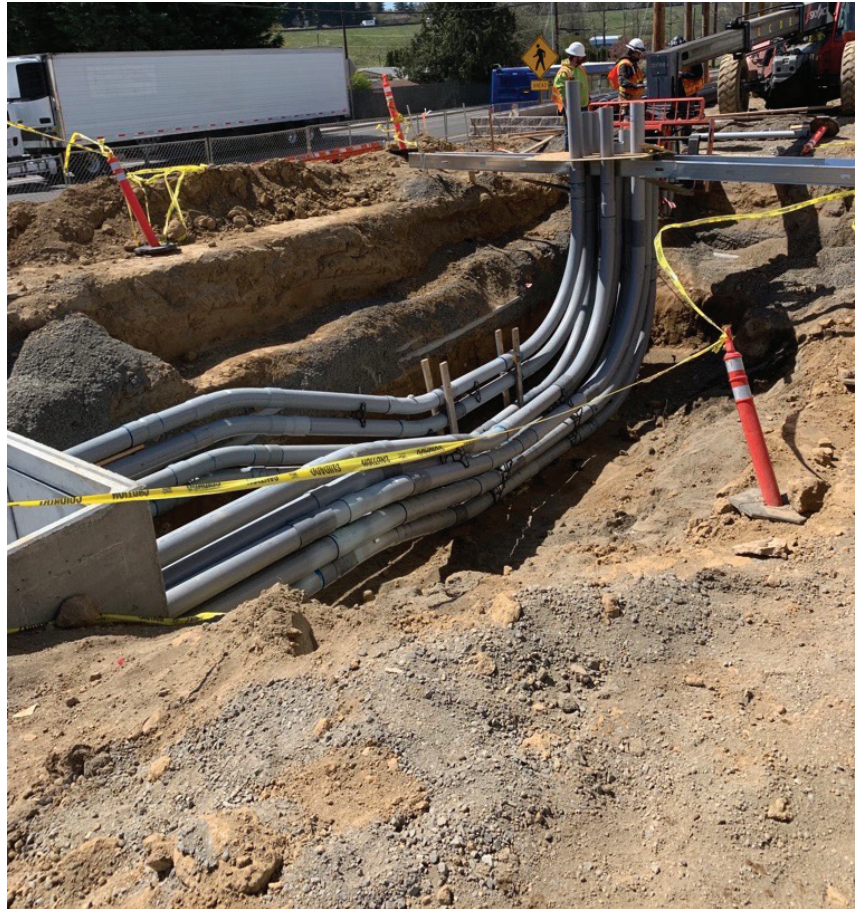
Figure 24. Backfill Required under Conduits
