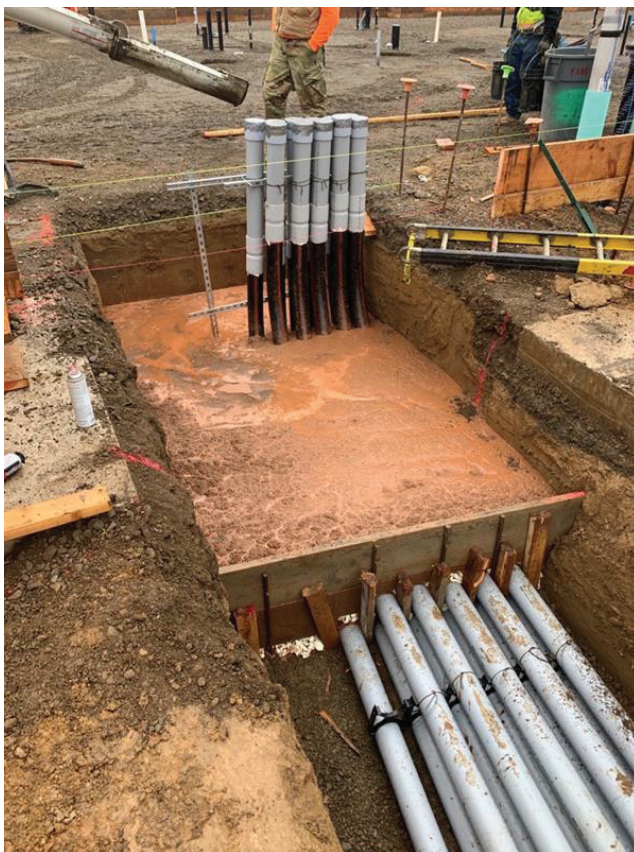
Figure 31. Plant-mixed Red Dye is Required when CDF or Concrete is Used
