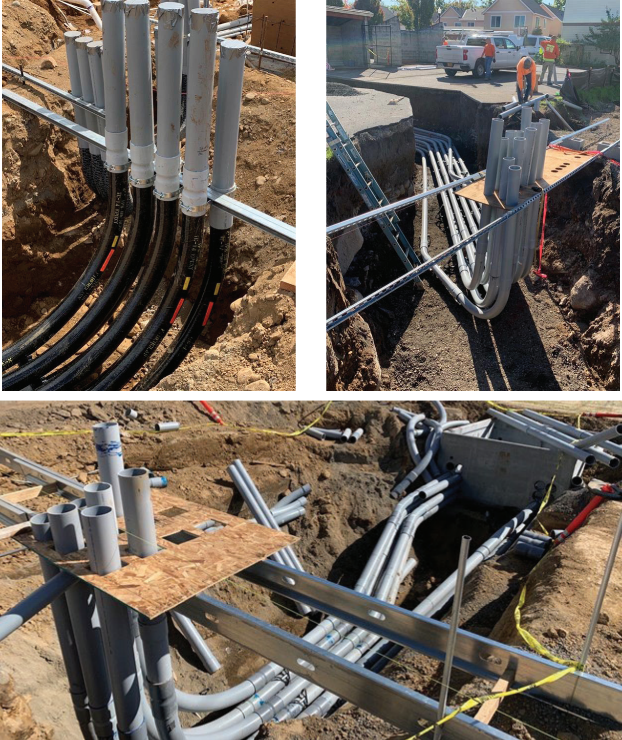
Figure 30. Spacers for Conduit Installed in Switchboards
