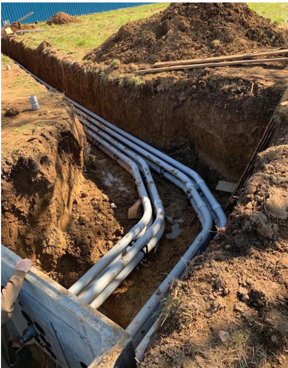
Figure 22. Conduit Exiting Vault with 3 Feet Straight Distance
