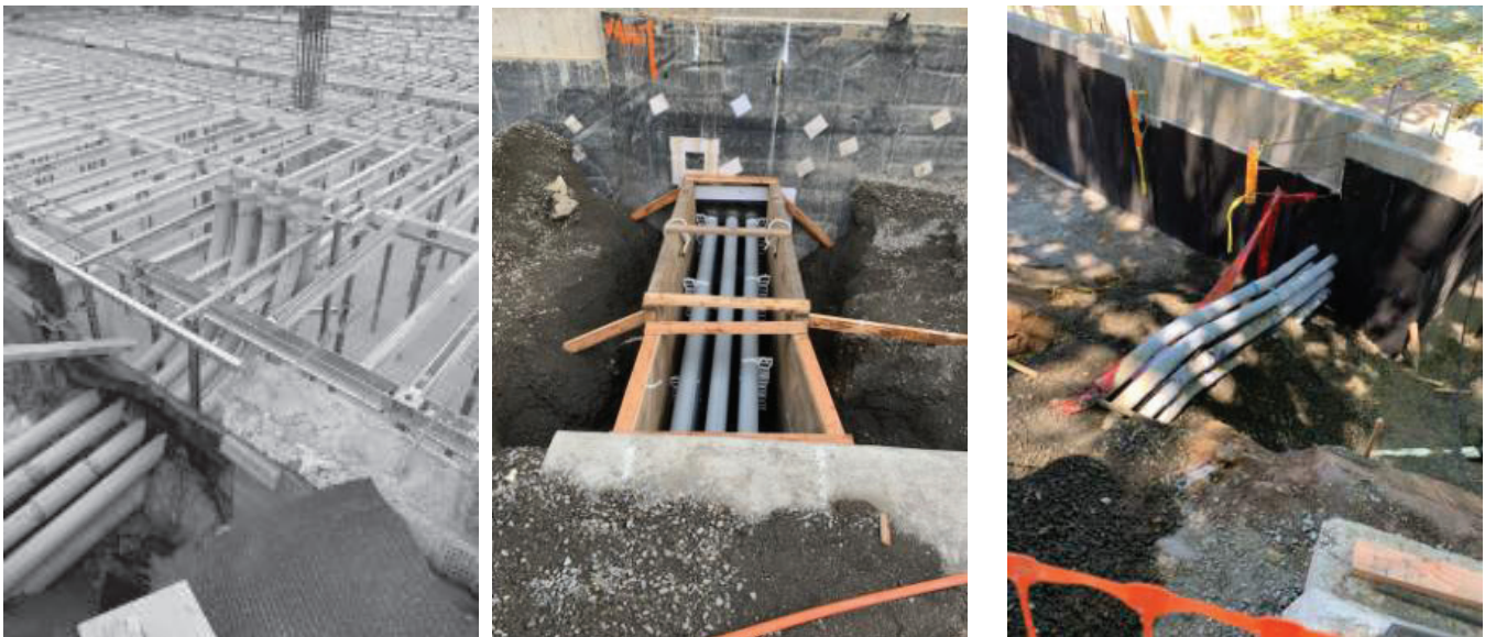
Figure 26. Conduit Routing/Alignment into Buildings
