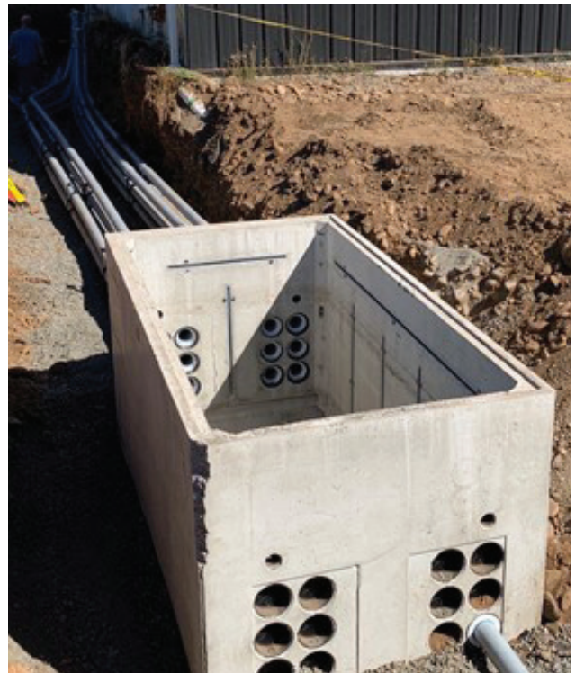
Figure 23. Conduit Termination Reducers
