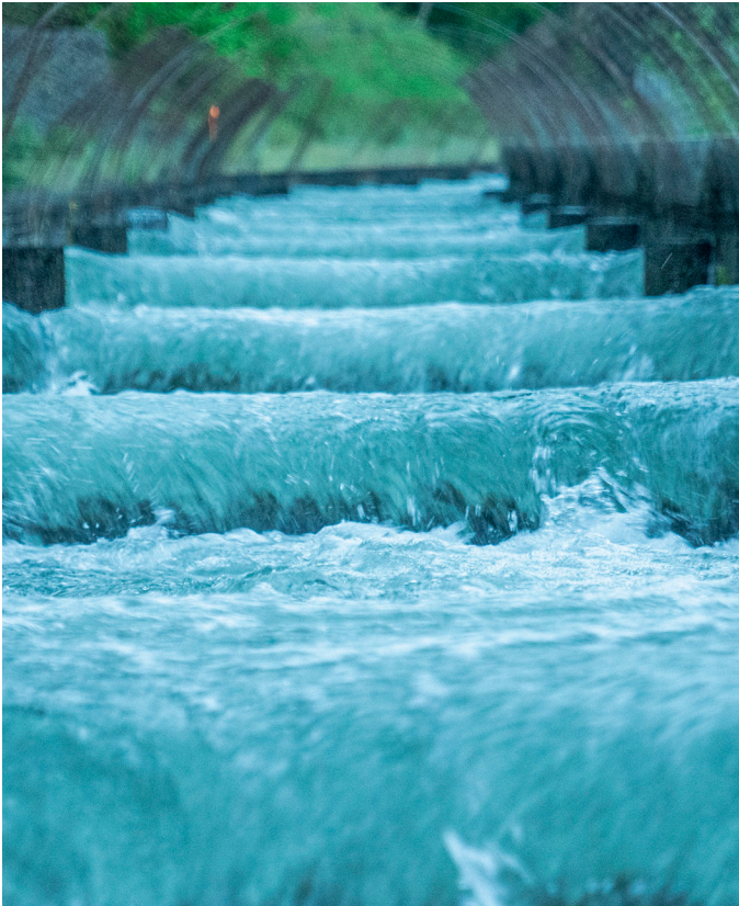
PGE’s North Fork Hydroelectric Plant outside of Estacada, OR
