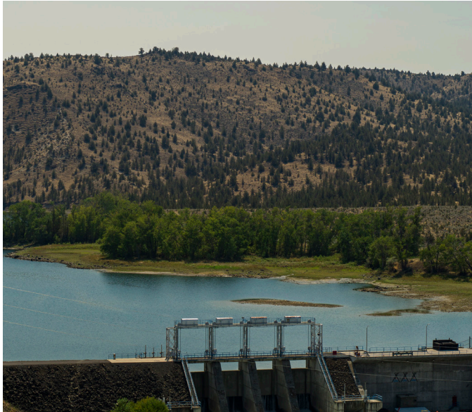
Pelton Round Butte Hydroelectric Complex near Madras, OR
