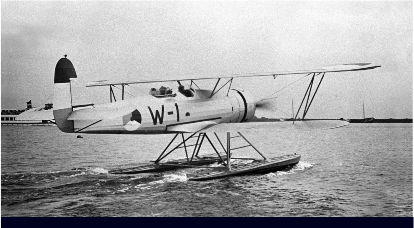
*The W-1 prototype is ready for a test flight. During testing, some edges of the fuselage panelling were taped over as a precautionary measure. The prototype featured a Scarff ring in the rear cockpit. (Collection: N. Braas)*
