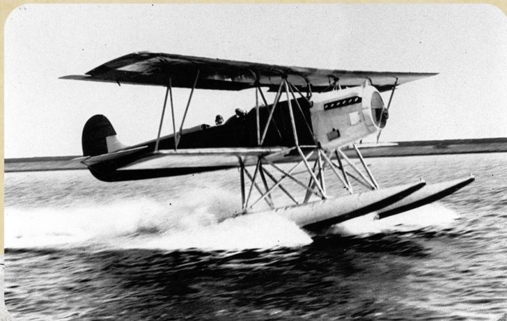
Following the B.II, Fokker reverted to modifying the successful Fokker C.V reconnaissance plane. It featured a revised and strengthened float gear yet suffered structural issues leading to cancellation of the project.
