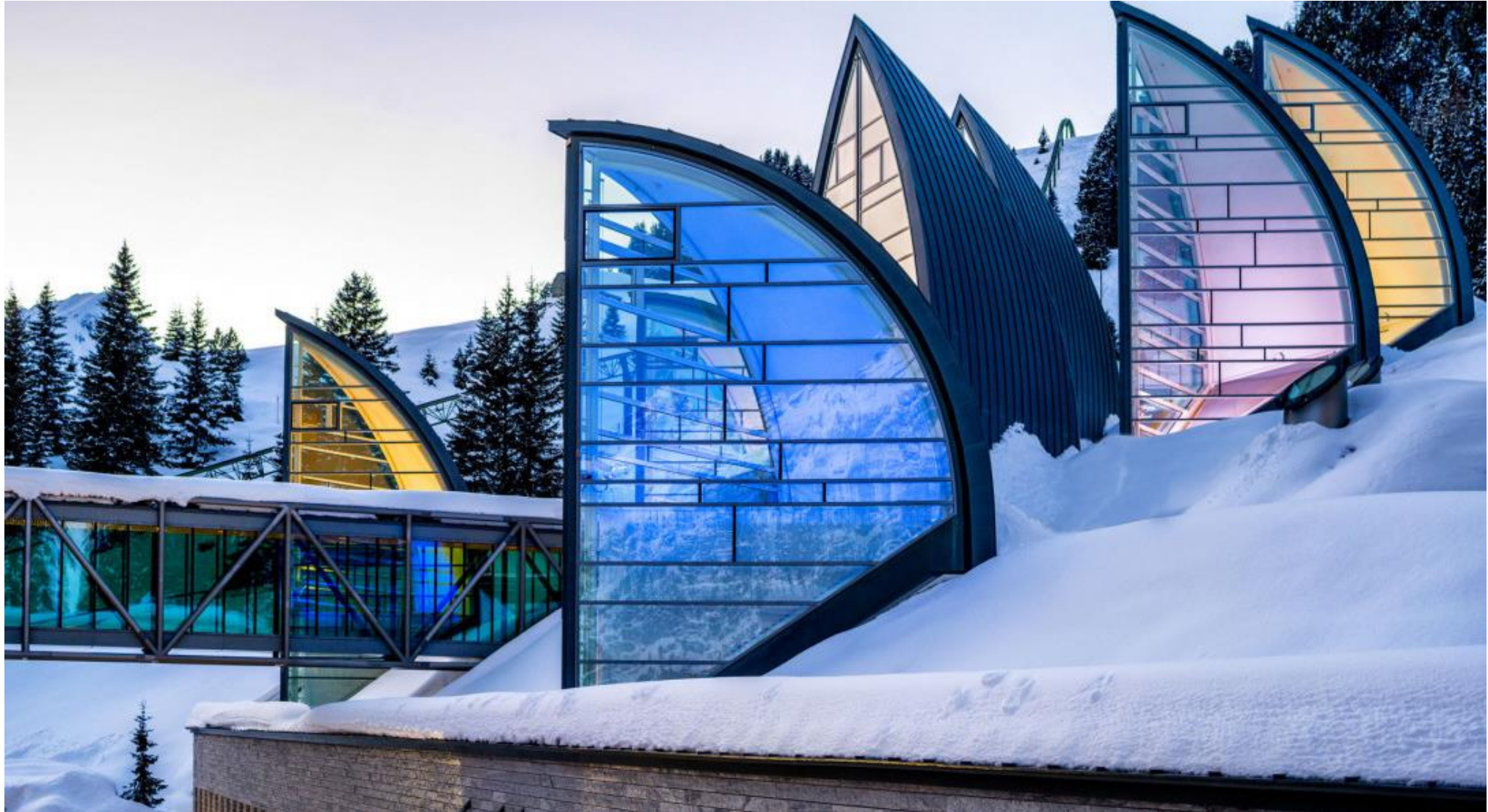
BERGOASE SPA – TOPPED BY ITS FUTURISTIC LIGHT TREE WINDOWS
