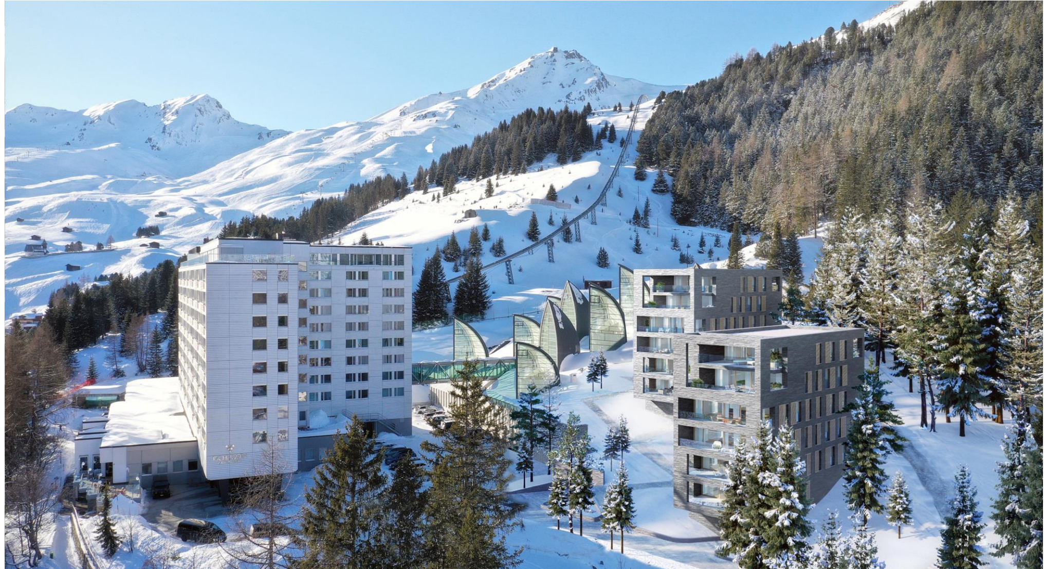
NEW MOUNTAIN LOFTS
