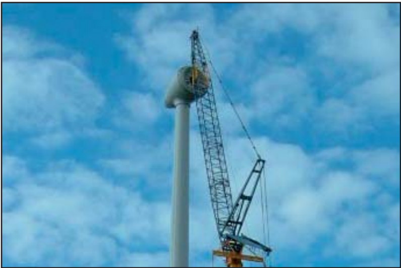
Photo F: Nacelle and hub are connected to the tower section
