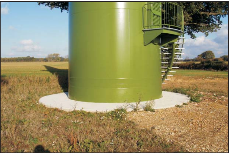
Photo D: Concrete flange
