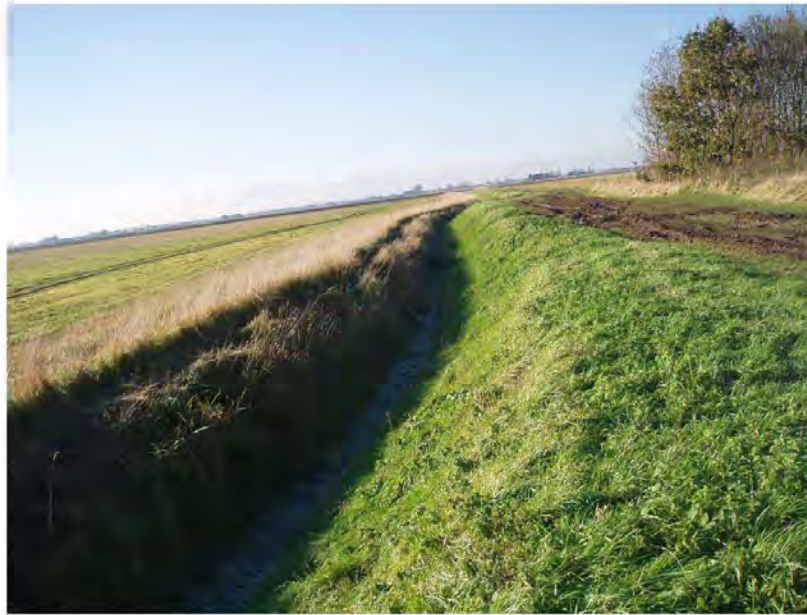
Figure 1 Typical small field drainage channel. Depth approx 2m below ground level
