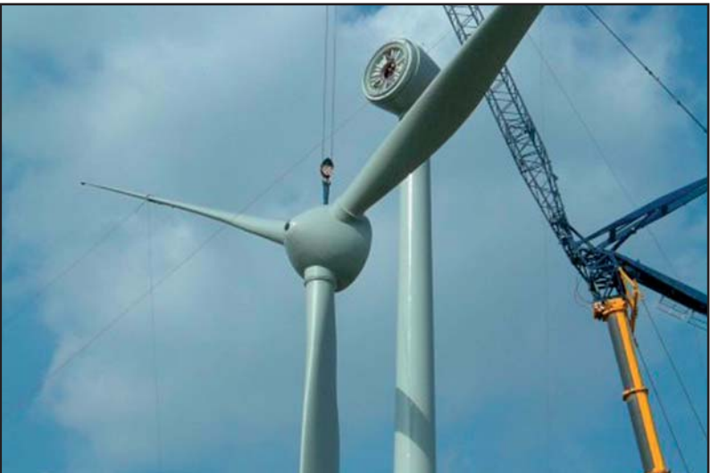
Photo G: Both hub and blades lifted together for connection to the nacelle
