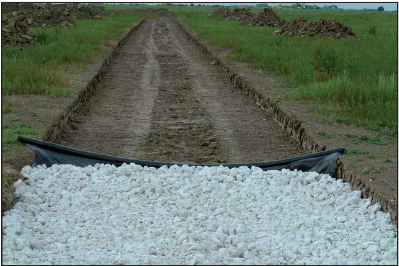
Photo B: Construction of access track
