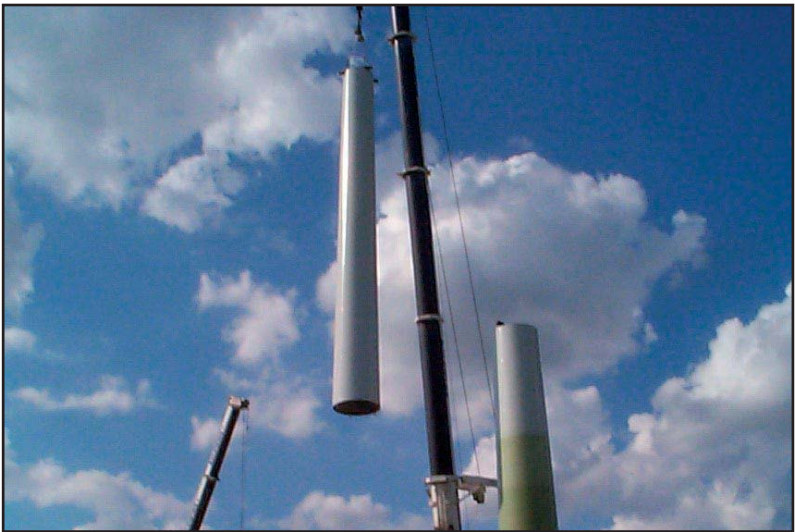
Photo E: Second tower section being lifted into place
