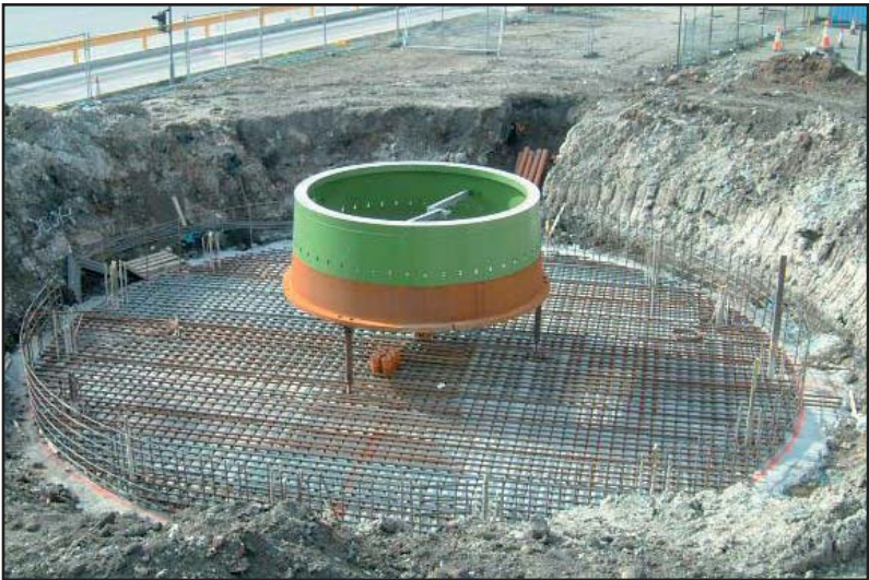
Photo C: Turbine foundation
