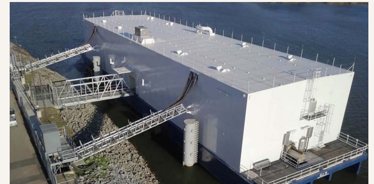
Nautilus Data Center
