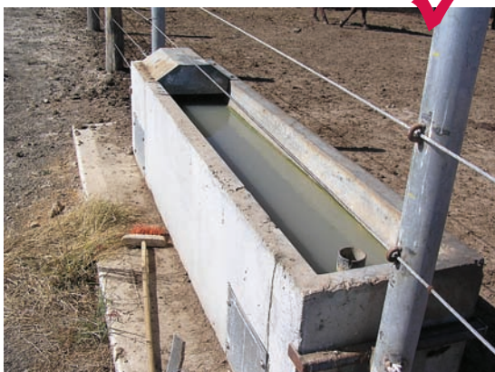
Good float protection, enclosed sides, overflow pipe and brush for cleaning.
