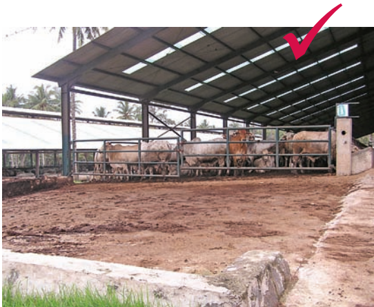
Clear-span structure, with good pen slope.
