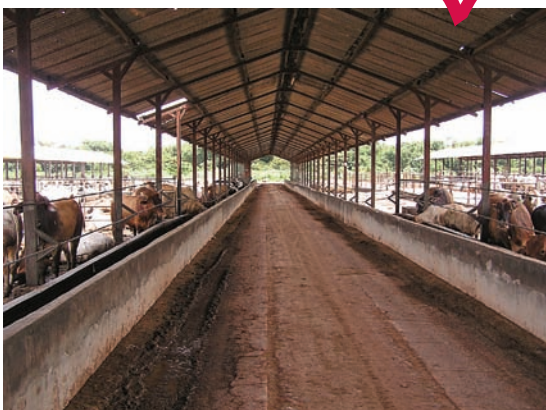
Wide feed alley gives clear access to troughs for feed delivery vehicles.
