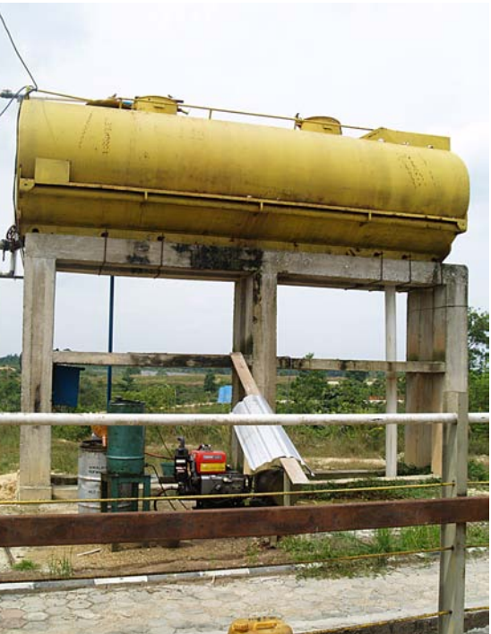
Raised water tanks can supply essential water even when power is cut.
