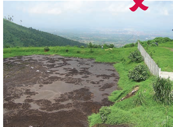
Poor sedimentation performance overloads pond with solids.
