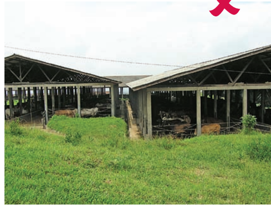
Sheds too close, and no ridge vents; poor natural ventilation.
