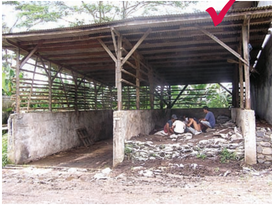
Fully covered bunk stockpile provides good protection from moisture.
