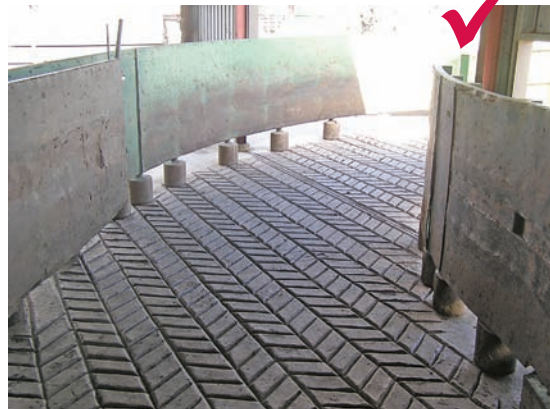
Grooved pattern on concrete ramp floor prevents cattle from slipping.
