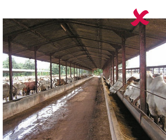
Insufficient cover to prevent rain entering shed and spoiling feed.
