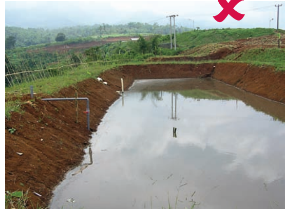
Unlined effluent storage ponds can cause pollution of groundwater.
