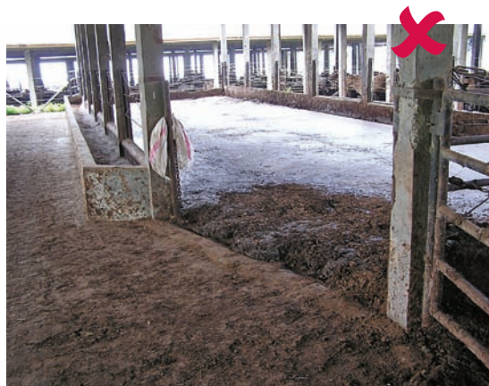
Pen overdue for cleaning and fresh bedding.
