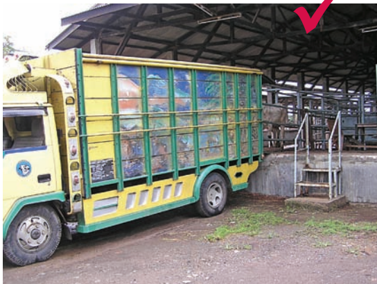
Clear access for trucks to loading/unloading ramp. Working area fully covered.
