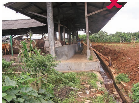
Narrow feed alley prevents delivery of feed by vehicle.
