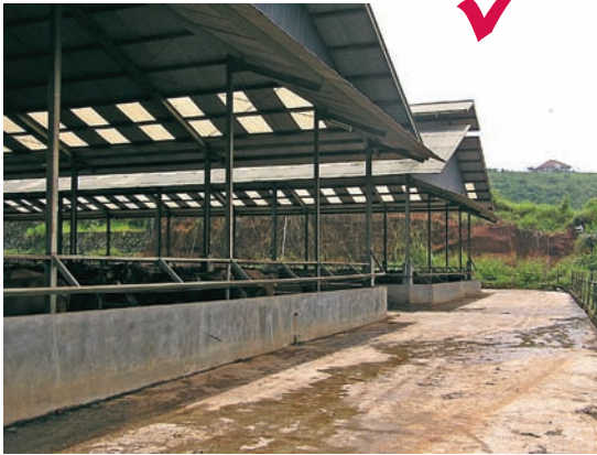
High eaves, good roof pitch and raised open ridge vent.
