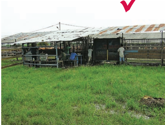
Covered working area protecting weighing box, crush and drafting gates.
