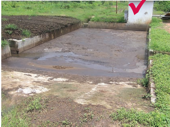
Well-maintained trafficable sedimentation structure effectively removes solids.
