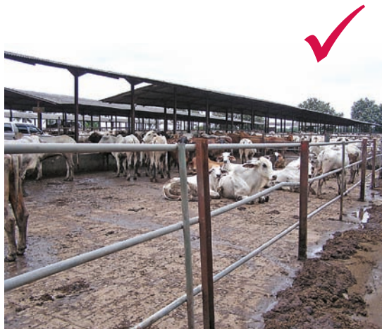
Stamped concrete to prevent cattle slipping in uncovered pen.
