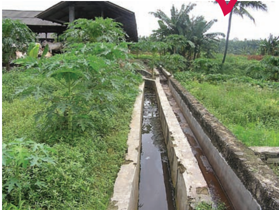
Raised edges on drains exclude clean water runoff from effluent system.
