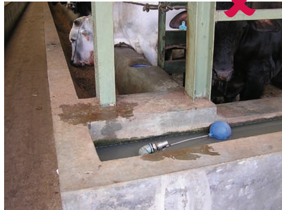
An exposed float valve can be easily damaged.
