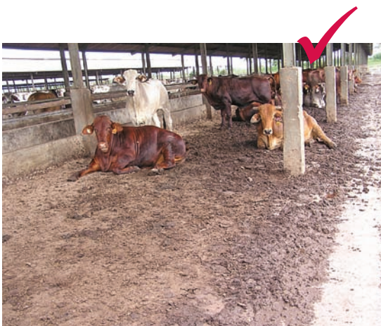
Sufficient cover for cattle and feed, and concrete encased columns.
