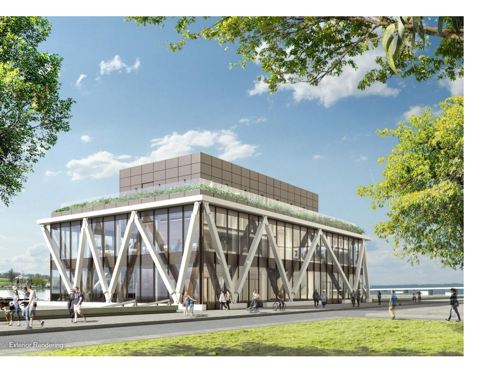
Part of the new District Wharf community in Washington, D.C., this building is designed as a beacon that offers a new waterfront gathering place for the city. By lifting the building above the water on a series of concrete piers, our design opens up commanding views down the Washington Channel towards the Jefferson Memorial. To eliminate the need for a column grid, we suspending the building from its truss-work, maximizing flexibility and creating vast and airy interior spaces.
