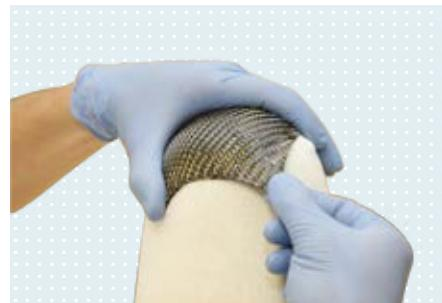
Position the tailored carbon fibre sections on those parts of the reinforcements that are to be strengthened while pre-tensioning them in the fibre directions.
