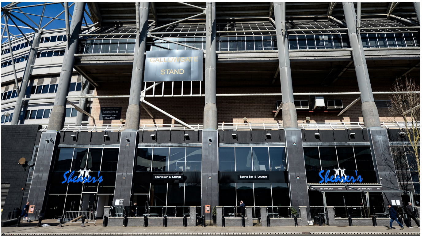
Figure 22. Ramp into 'Shearer's Sports Bar' with assisted entry doors
