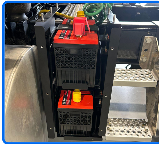
Example image: Additional batteries behind driver's side fuel tank (uncovered); International
