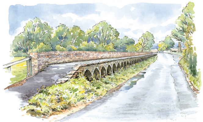
Kellaways Arches, 1812 Sixty-four stone arches were built to cross flooded fields
