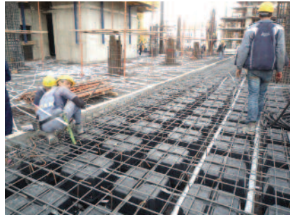
FORMWORK BETWEEN U-BOOT SLAB AND SOLID SLAB
