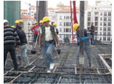
DIFFERENT PHASES OF CASTING A U-BOOT SLAB
