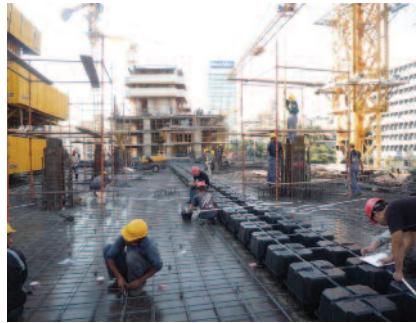
INSTALLATION OF U-BOOT ELEMENTS
