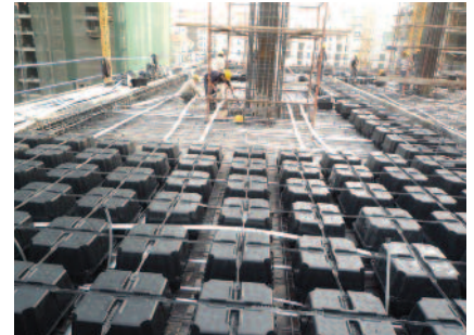
INSTALLATION OF DUCTS FOR POST TENSIONING WITHIN THE U-BOOT SLAB
