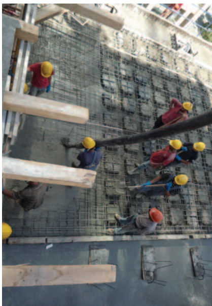
DIFFERENT PHASES OF CASTING A U-BOOT SLAB
