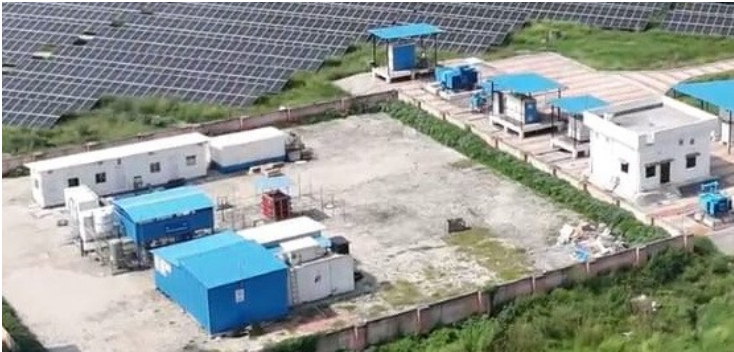
Fig. 5. Site photograph of the hydrogen microgrid.
