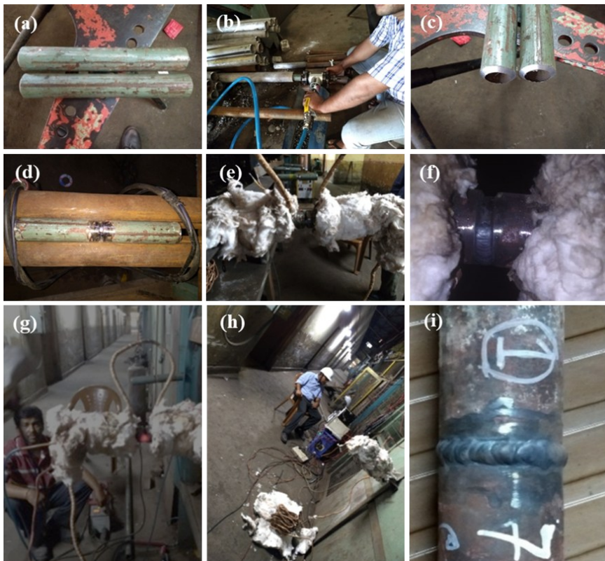
Fig 1. Photographs showing different stages of Welding of T91 Boiler Tubes. (a) Cut to Length, (b) Face or Bevel, (c) Cleaning, (d) Alignment, (e) Root Pass, (f) Hot Pass, (g) Heating Cycle in PWHT, (h) Soaking and Cooling Cycle and (i) Final Welded Tube
