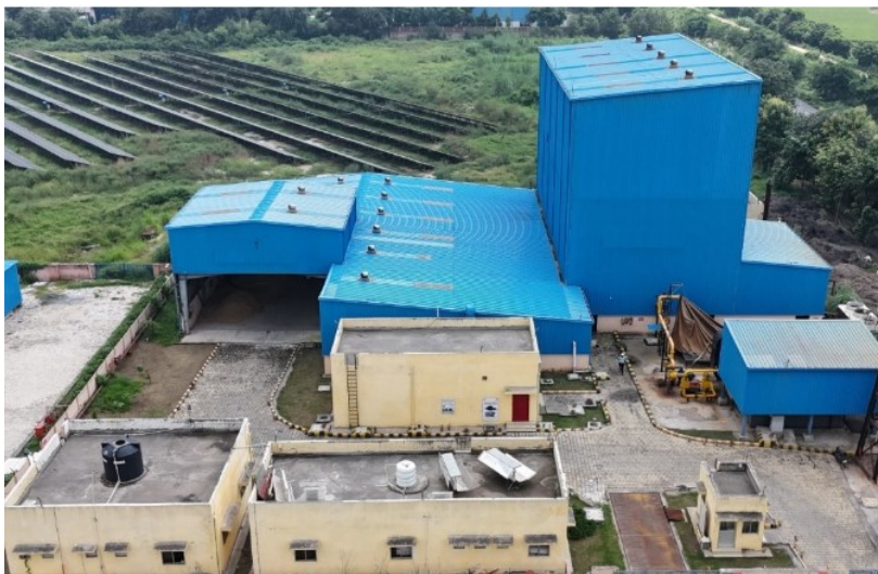
Fig. 3. Photograph of the RDF gasification-based net 400 kW X 24 hrs power generation plant.
