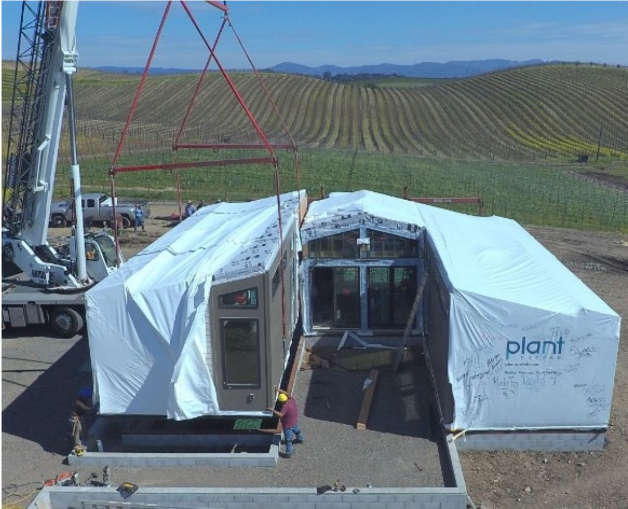
Modules are wrapped before departing the factory. On installation day (above), the hinged roof is visible beneath the plastic wrap, flipped onto the main roof along the exterior walls.
