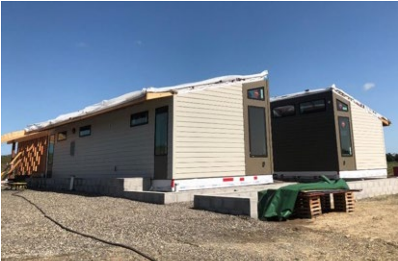
Post-installation, modules are attached to the foundation and the roof is flipped into position.
