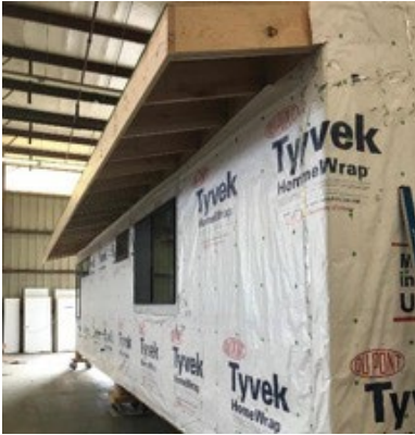
In the factory, the roof is constructed with overhang and then flipped onto main roof for shipping.
