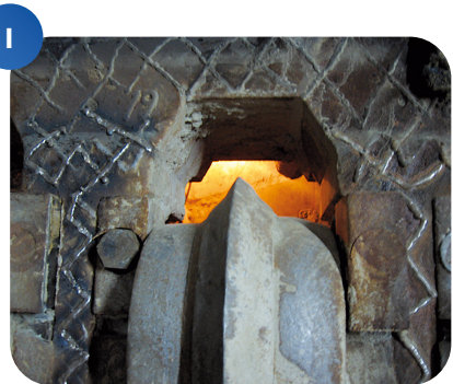
1. Anti-wear and anti-dust: MasterRoc® ABR 5 / Anti-dust: MasterRoc® ABR 2 and 7
