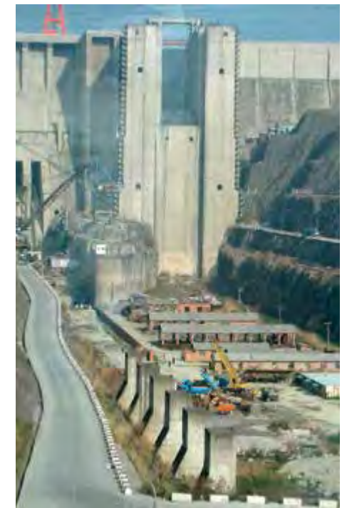
New ship's lift, Three Gorges Dam, Yangtze River
