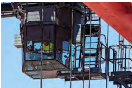
Gantry crane driver cabin
