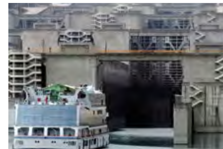
Locks on the Three Gorges Dam, Yangtze River
