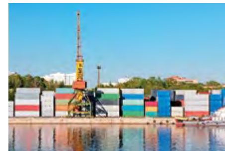
Container terminal in Moscow
