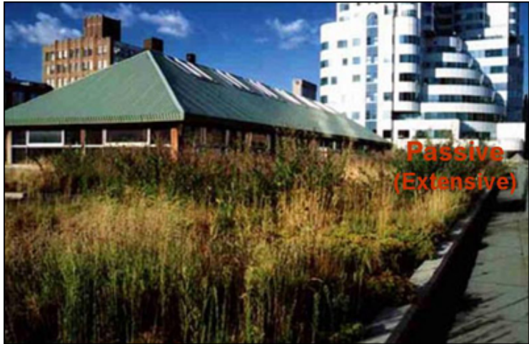
Figure 7. The Mountain Equipment Co-op green roof was built in 1998, and uses a shallow garden medium (City of Toronto, 2011a).
