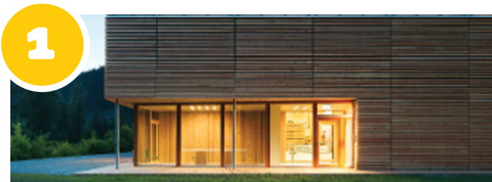
BC Passive House Factory
