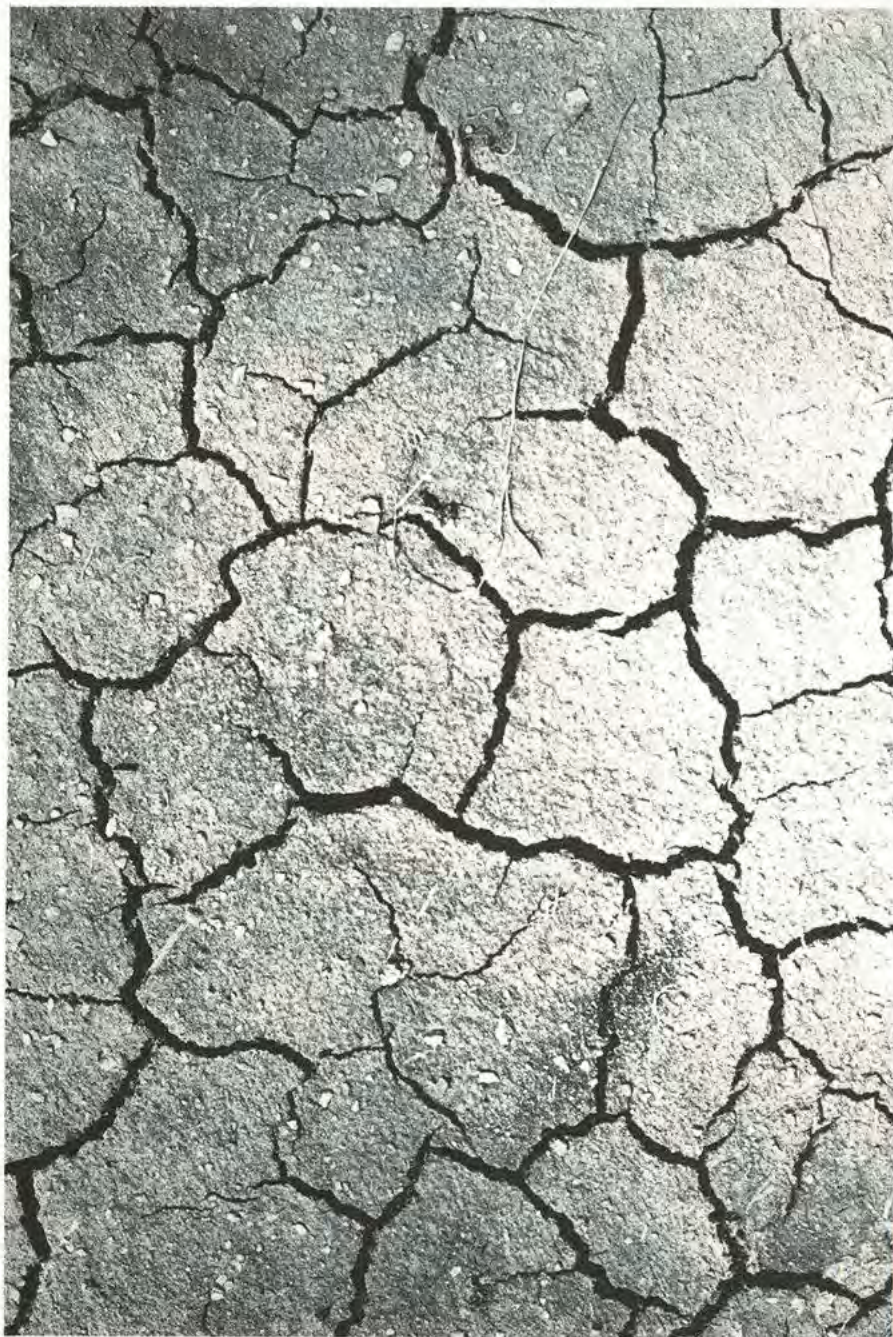
Expanding Soils & Their Effect on Underground Pipe
