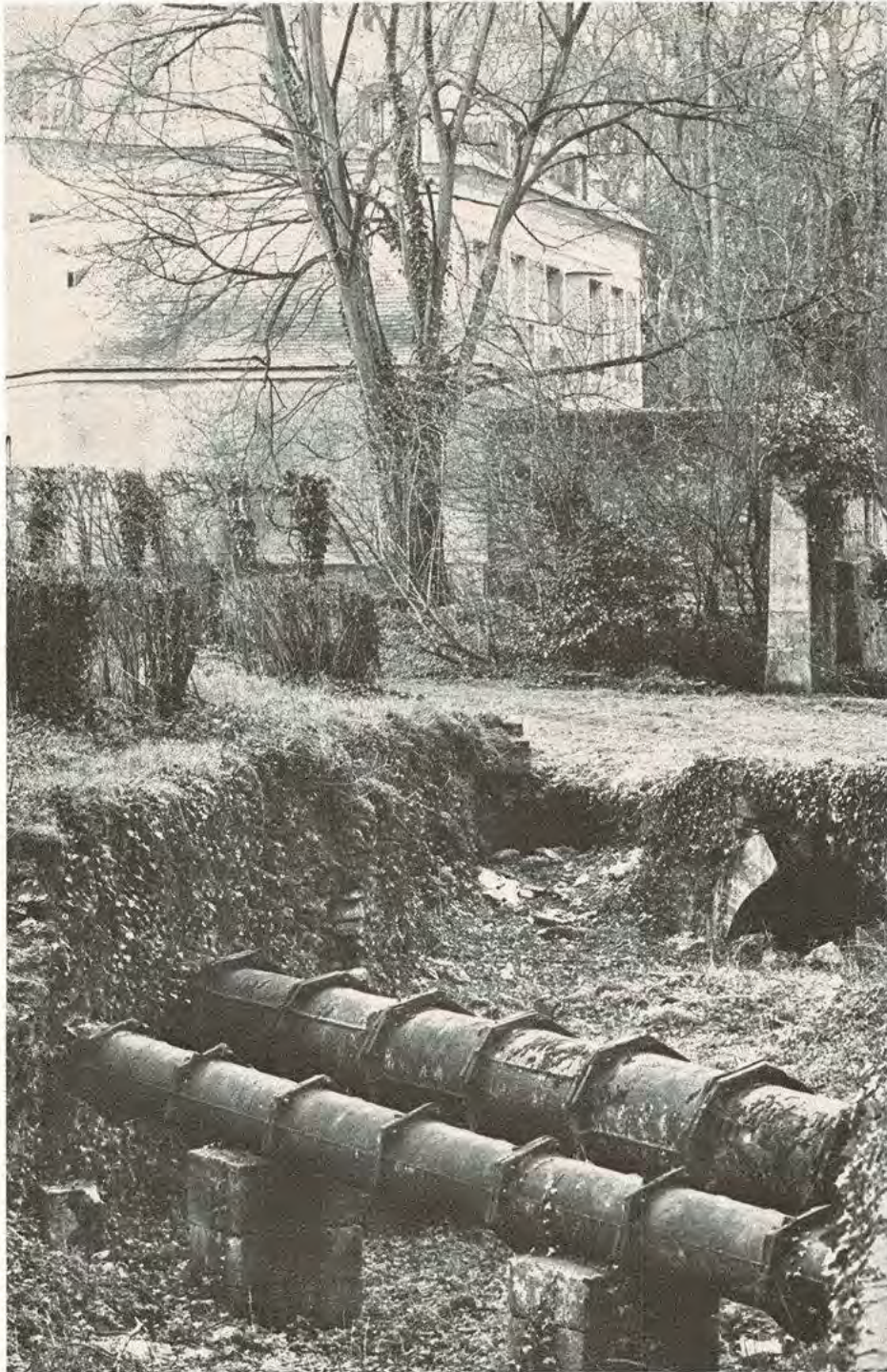
Cast Iron Pipe Installed 1664 Versailles
