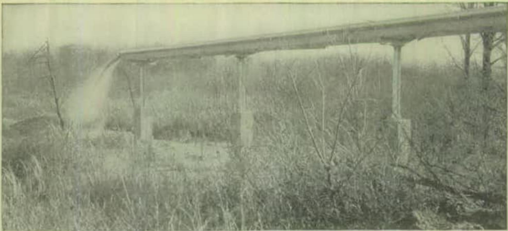
Steam Generating Plants Cast iron pipe carries over 40 tons of ash daily in ash removal system.
