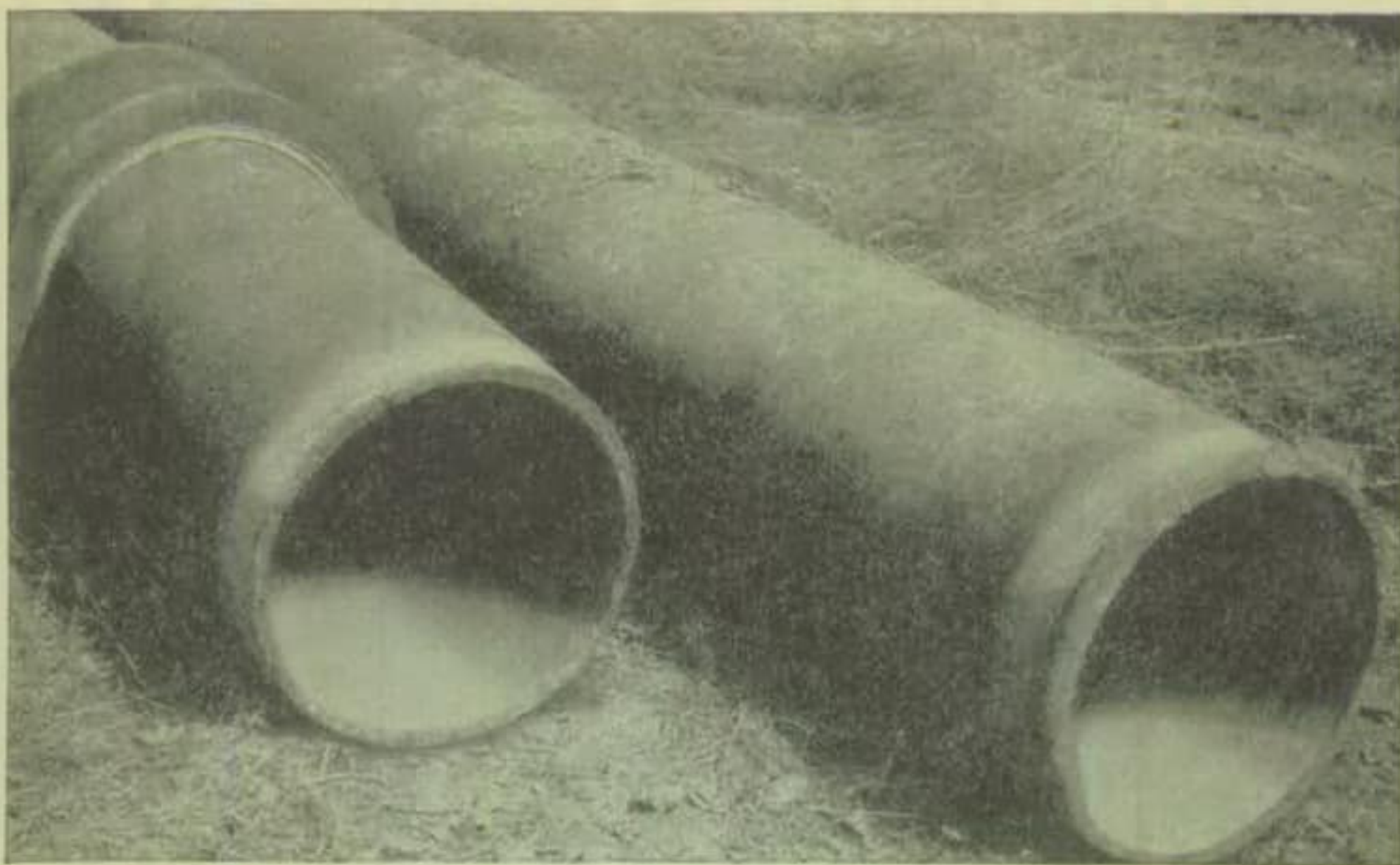
Springfield, Missouri. In connection with changes at a pumping station, part of a 50-year-old 18-inch cast iron water main was recently taken up and relaid in another part of the city. Note cast marks and date clearly discernible on pipe in right center.
