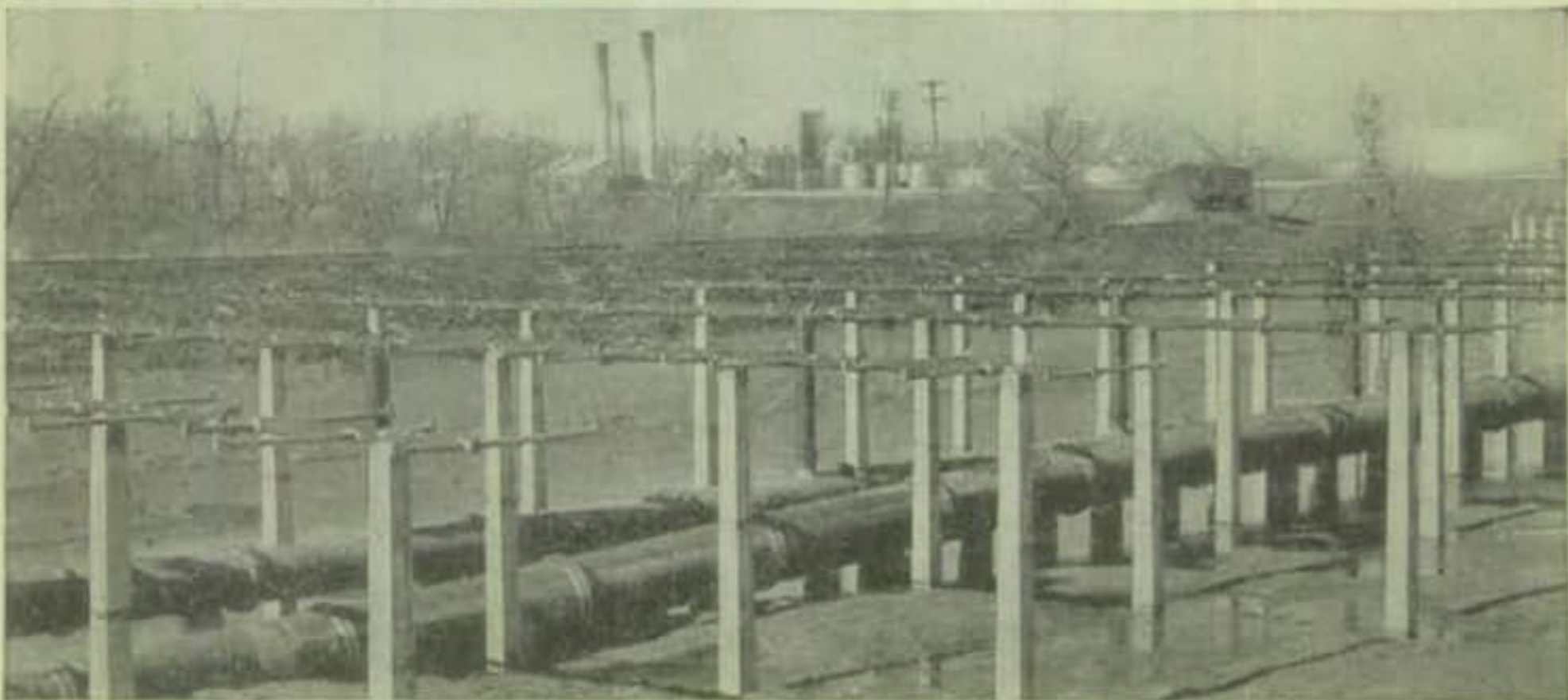
Oil Refineries Cast iron pipe installed for cooling coil.
