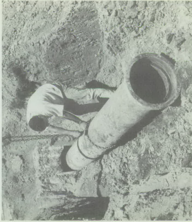
CHEEKTOWAGA, NEW YORK—39-year-old pipe; good as new! That's the comment of officials inspecting this 16-inch cast iron pipe that was placed in service in 1925, which was removed in 1965 to make way for new construction. Other cast iron pipe installed in 1901 at same site was inspected at same time, and tap sample proved it to be in excellent condition.
