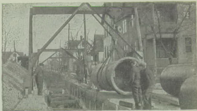
Special Gantry Crane for Laying Large Pipe
