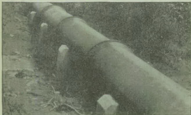
Pipe Supported on Concrete Piers
