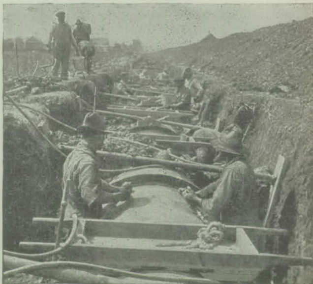
Pneumatic Calking with Lead Wool
