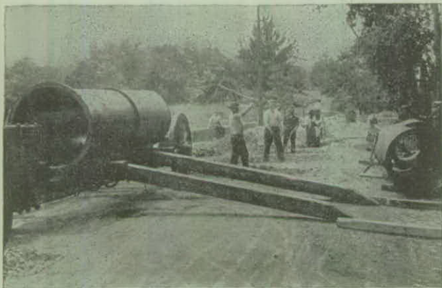
Unloading Pipe from Truck with Skids
