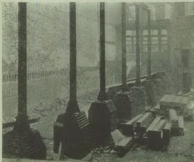
Cast Iron Pipe Columns Are Fire Resisting
