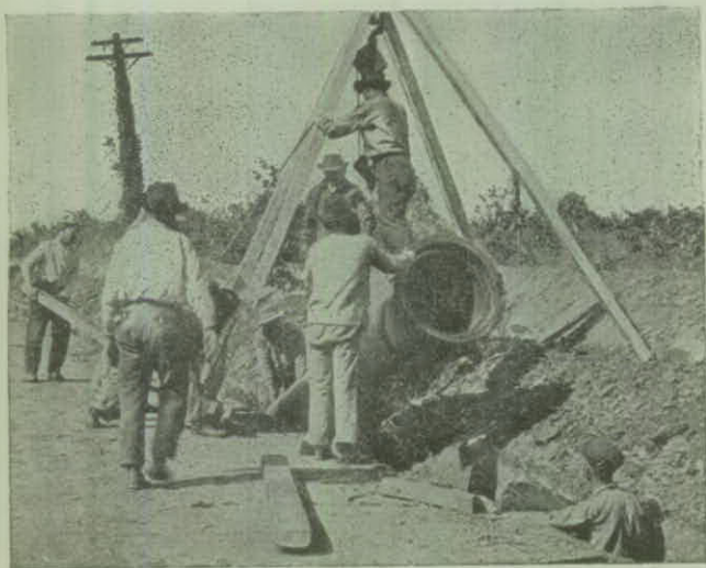
Tripod for Lowering Large Pipe into Trench
