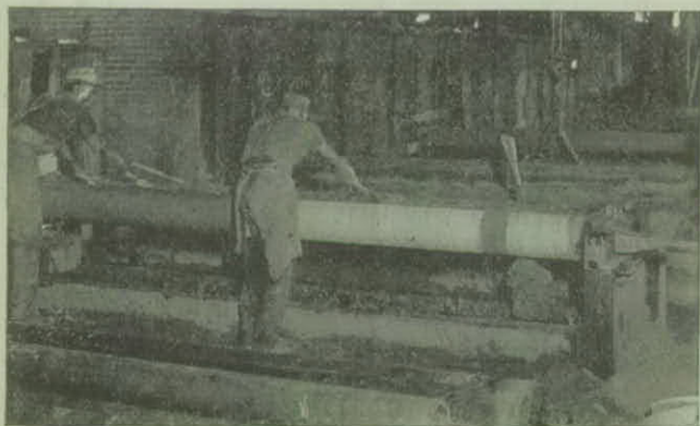
Core Making Showing Core Bar with Paper Wrapping
