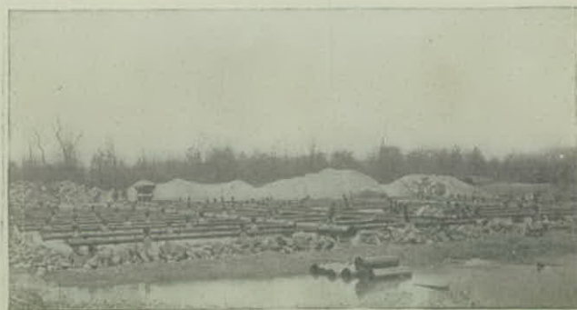
In a Sewage Disposal Plant
