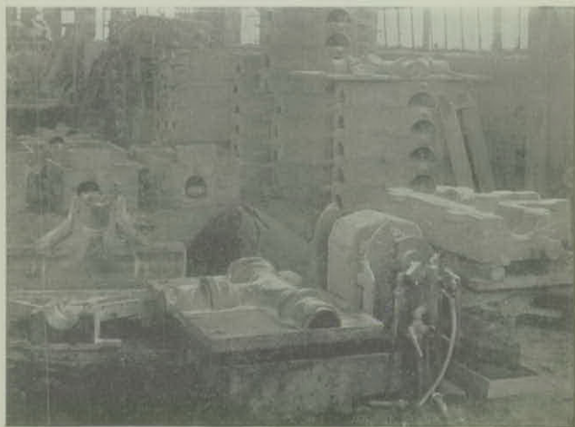
Molding Machine for Making Fittings
