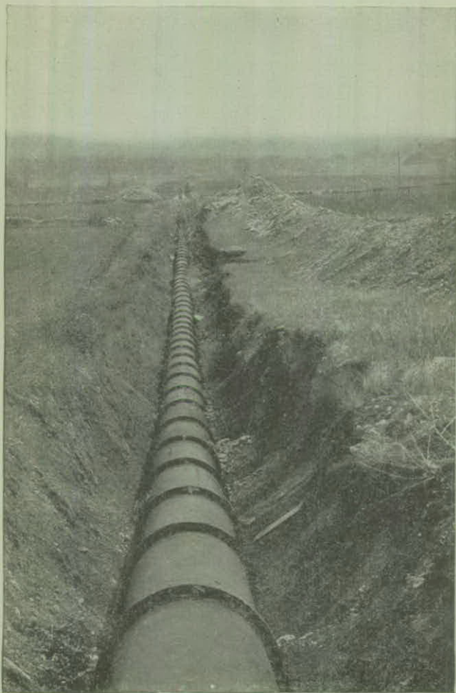
Long Water Supply Line Laid Through Rolling Country
