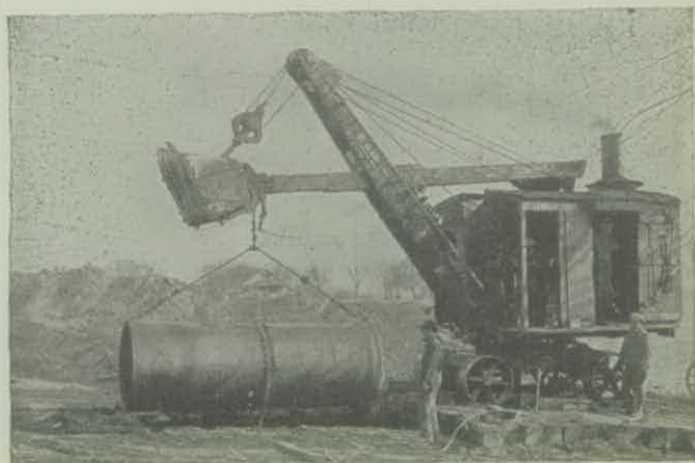
Handling Cast Iron Pipe with a Steam Shovel
