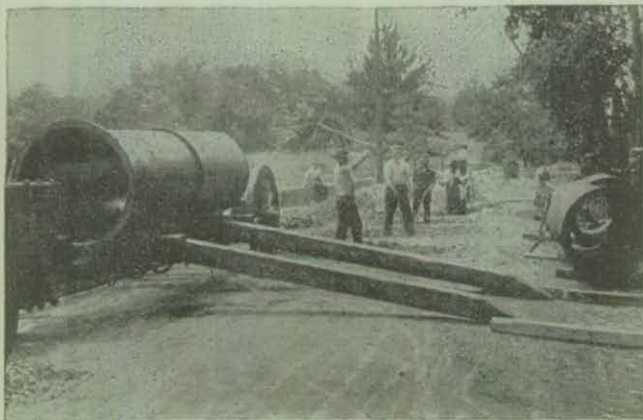
Unloading Pipe from Truck with Skids
