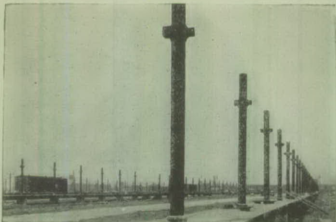
Cast Iron Pipe Columns in Warehouse Construction
