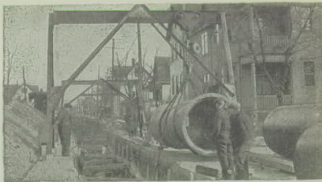
Special Gantry Crane for Laying Large Pipe
