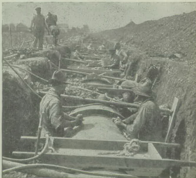
Pneumatic Calking with Lead Wool
