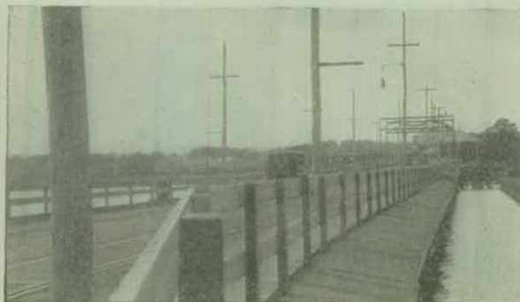
Wooden Protection Over a Pipe Line at Bridge Crossing
