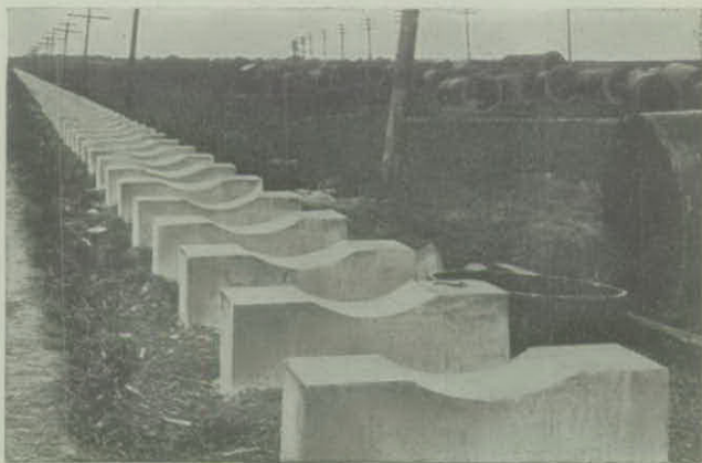
Concrete Piers to Support Pipe Through Filled Ground
