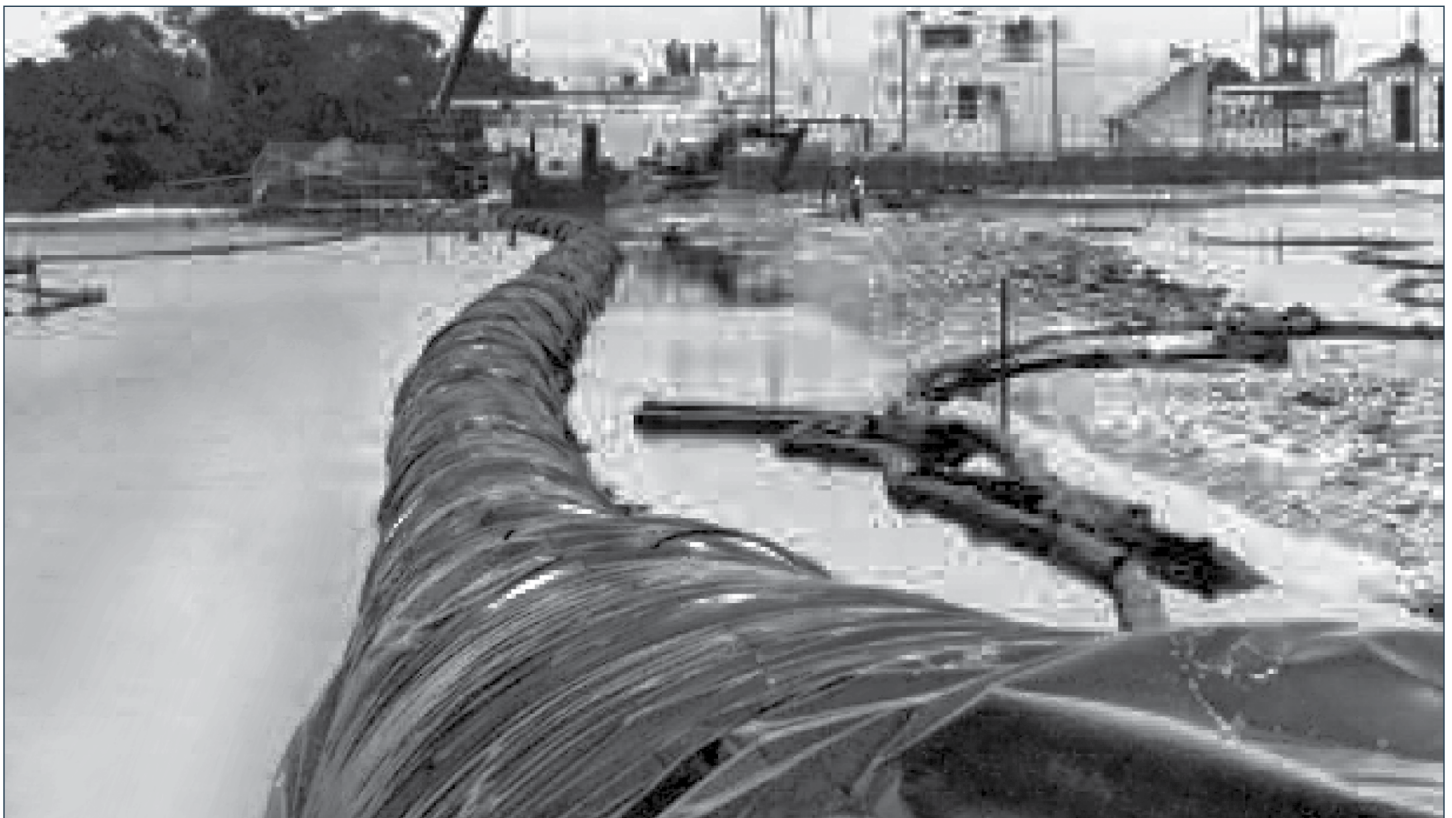
Polyethylene encasement can be used in some subaqueous crossings as corrosion protection for Ductile Iron Pipe.
