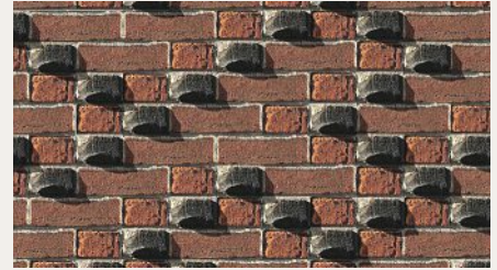
3 Built for a Baker, but which Scandinavian architect?
