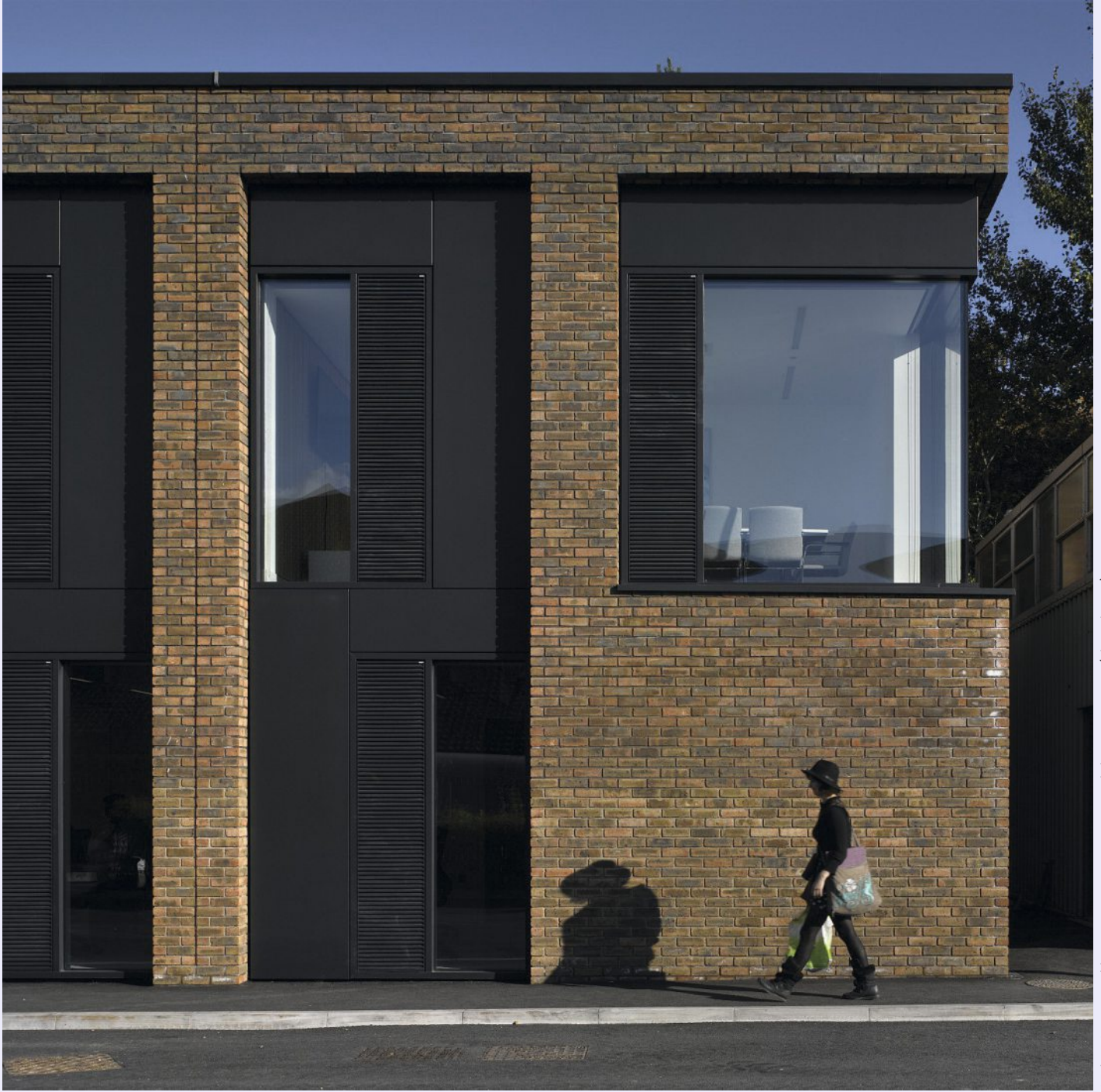
Student Services Building, Arts University Boumeimouth, by Design Engine (ph: Nick Kane)
